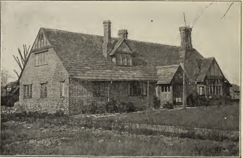
Fig. 89. — By decreasing the exposed length of shingles toward the top a greater apparent expanse is obtained.
