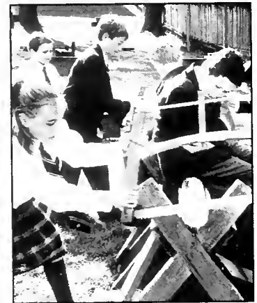
Fort Langley. Work dention has new meaning.
