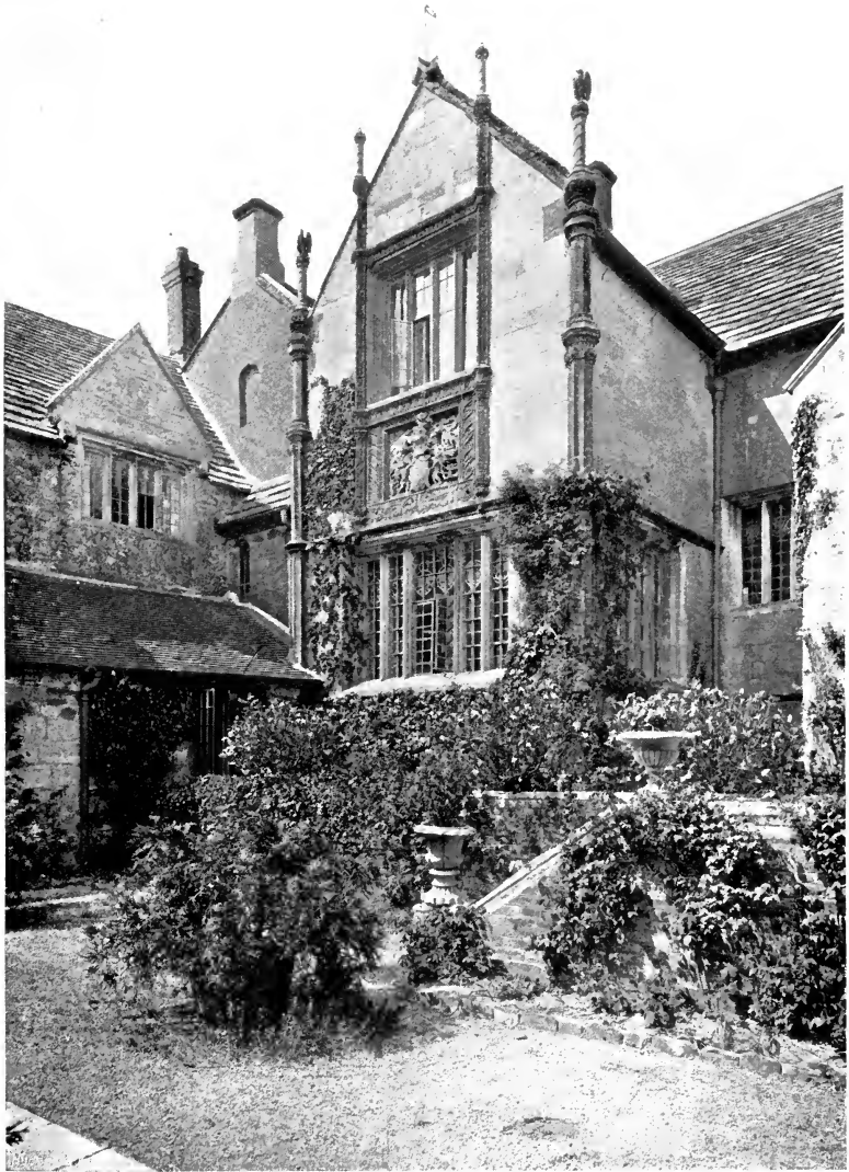
RESTRAINED USE OF CREEPERS ON AN OLD HOUSE THAT HAS BEAUTIFUL ARCHITECTURAL DETAILS.
