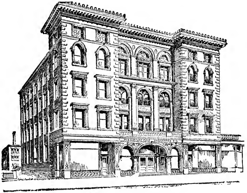
PIEDMONT INSURANCE BUILDING, SOUTH TRYON ST., CHARLOTTE, N. C. IN WHICH KING'S BUSINESS COLLEGE IS LOCATED
