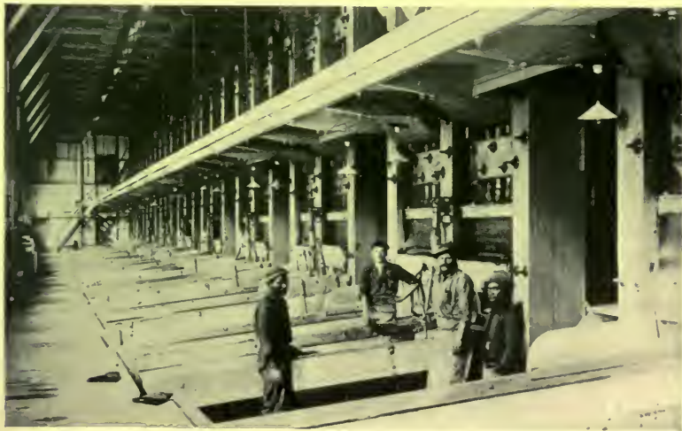
THE BATTERY, SHOWING THE MERCURY-COATED PLATES
