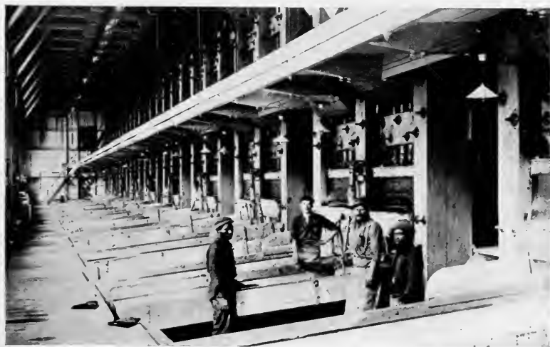
THE BATTERY, SHOWING THE MERCURY-COATED PLATES
