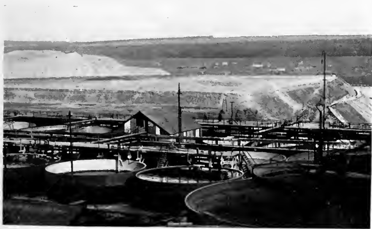
VIEW OF CYANIDE WORKS
