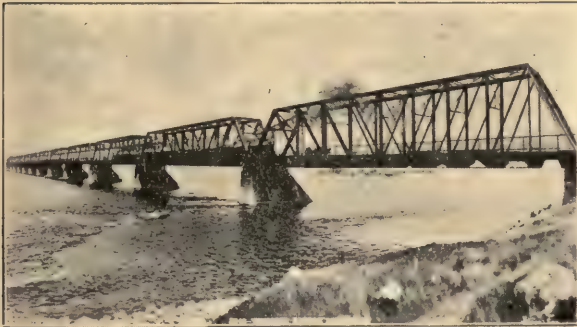
NEW VICTORIA BRIDGE.
