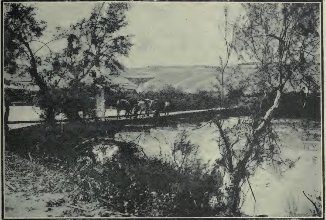
Pontoon bridge over the Jordan at El Ghoraniyeh.
