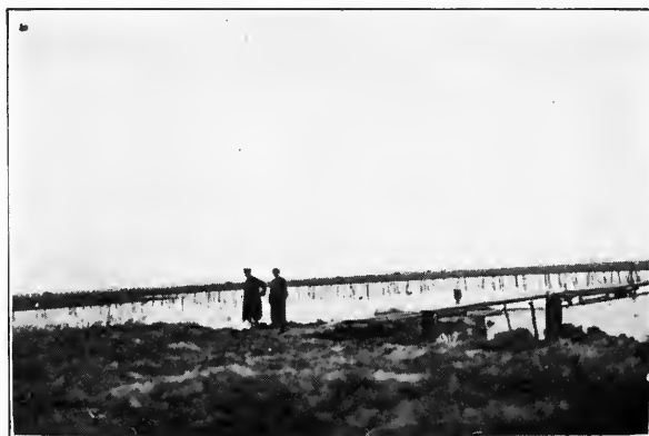
Between the Main and Front Line Trenches
