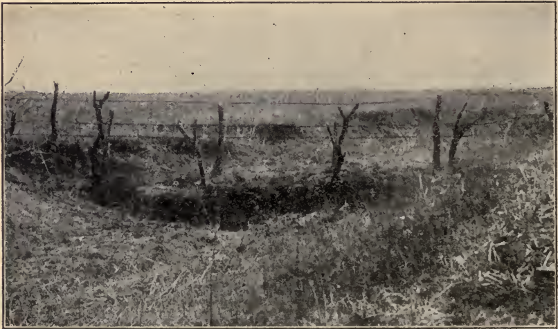
FIG. 20.—DAMS OF STRAW HELD BY WOVEN WIRE FENCING, MASON COUNTY
