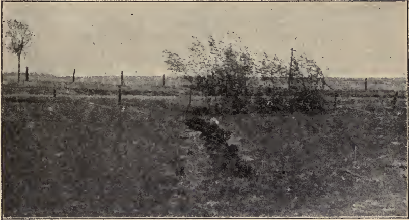
FIG. 8.—WATERFALL EROSION ON PASTURE LAND IN OGLE COUNTY
