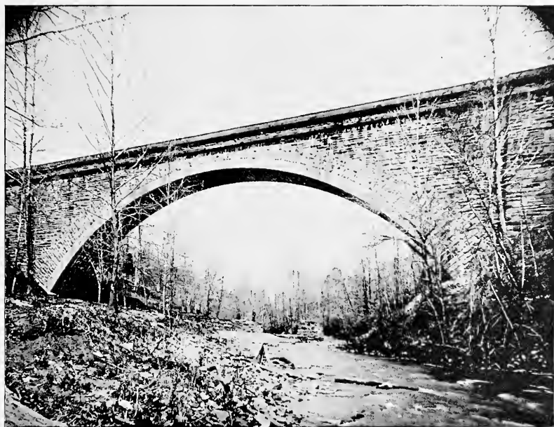
Cabin John Bridge, The Largest Stone Arch in the World. Span, 220 Feet
