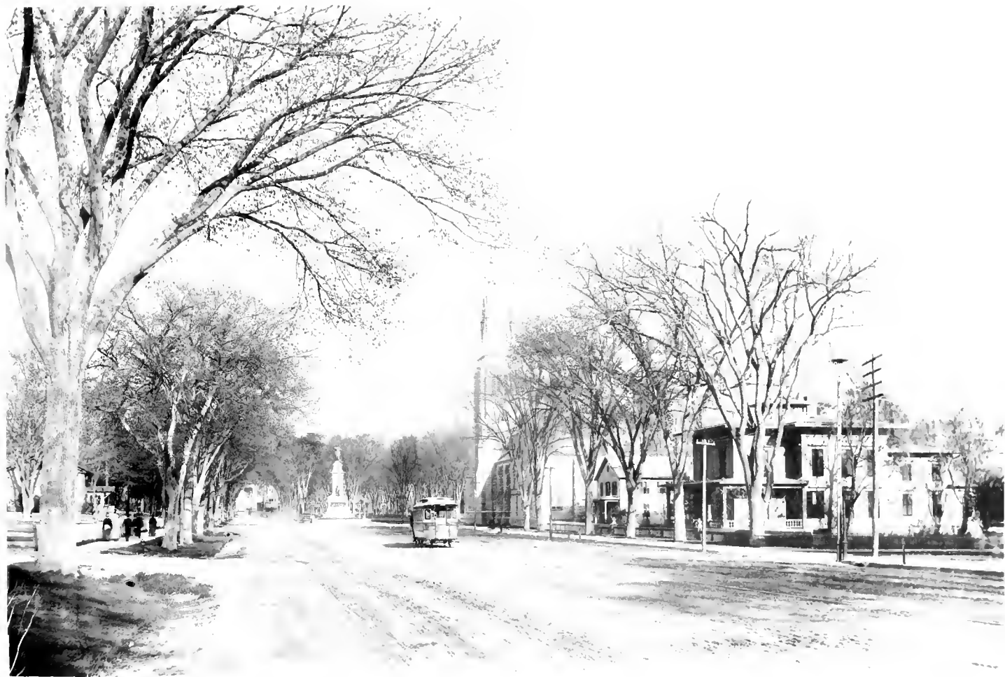
Market Street, New York Looking East
