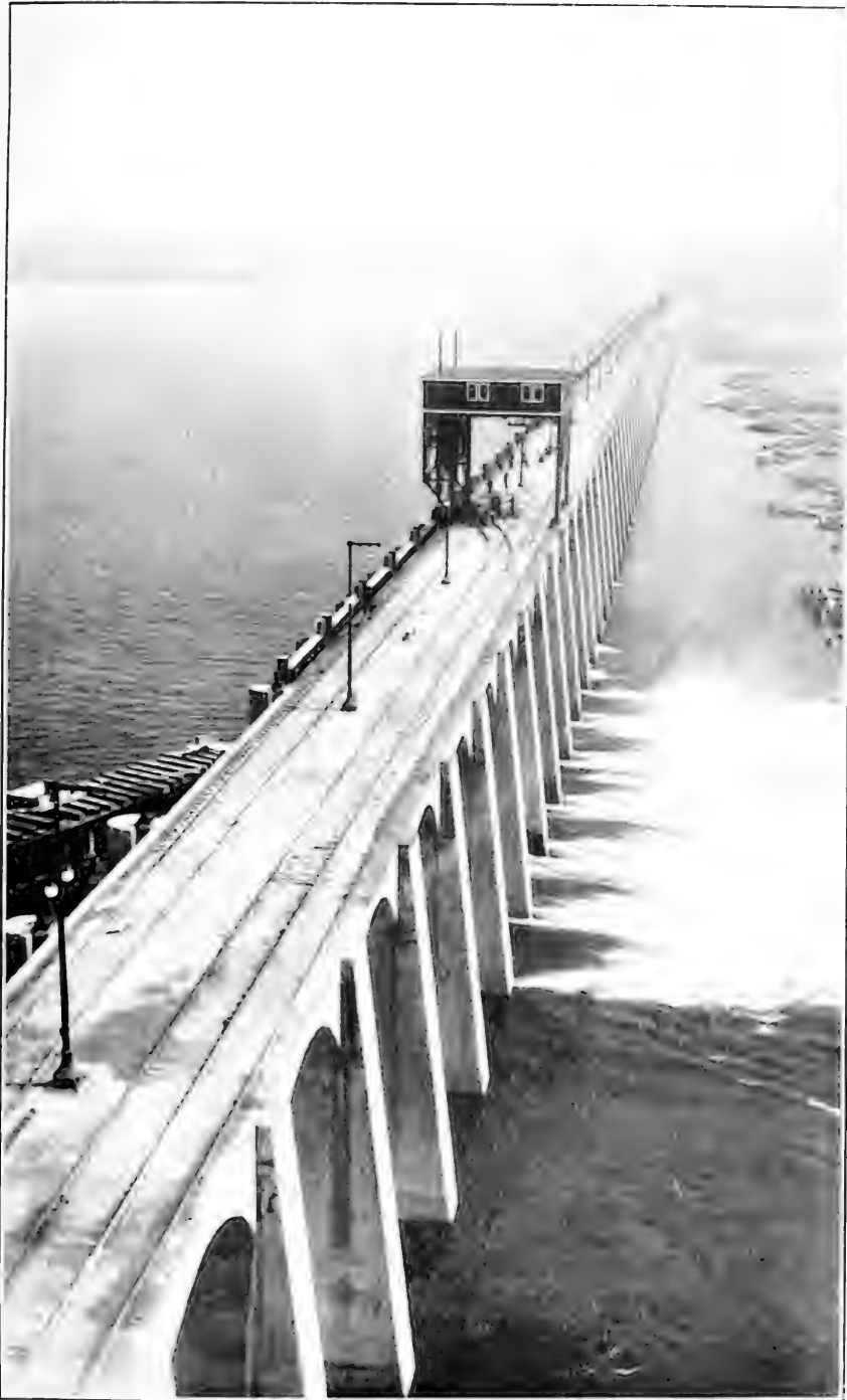
CONDITION BELOW THE DAM WITH SIX SPILLWAYS OPEN. NORMALLY A MUCH GREATER NUMBER OF SPILLWAYS ARE IN USE.
