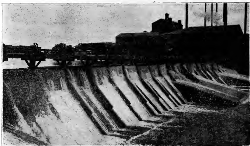
Fig. 377.—Adjustable Flash Boards at Eau Claire, Wis.
