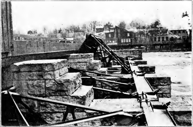
Fig. 373.—Tainter Gates at Lower U. S. Gov. Dam, Appleton, Wis.
