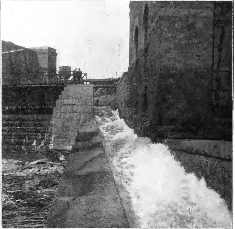
Fig. 387.—Log Way at Lower Dam, Minneapolis, Minn.
