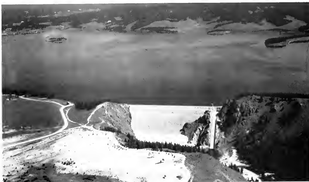
Granby Dam and Reservoir
