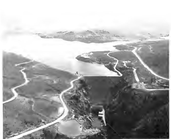
Blue Mesa Dam, Powerplant, and Reservoir
