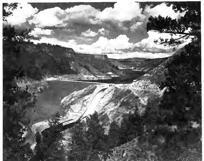
Anderson Ranch Dam and Powerplant
