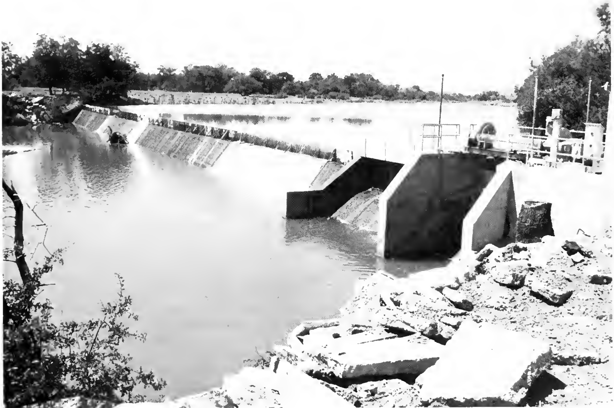
Northside Diversion Dam
