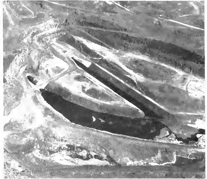
Outlet of Bacon Siphon and Tunnel
