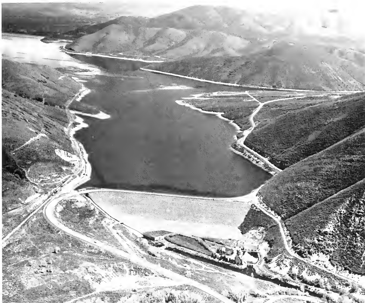
Deer Creek Dam and Reservoir
