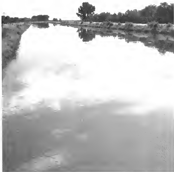
North Side Canal
