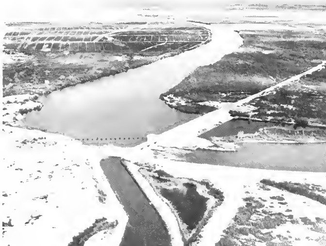
Palo Verde Diversion Dam
