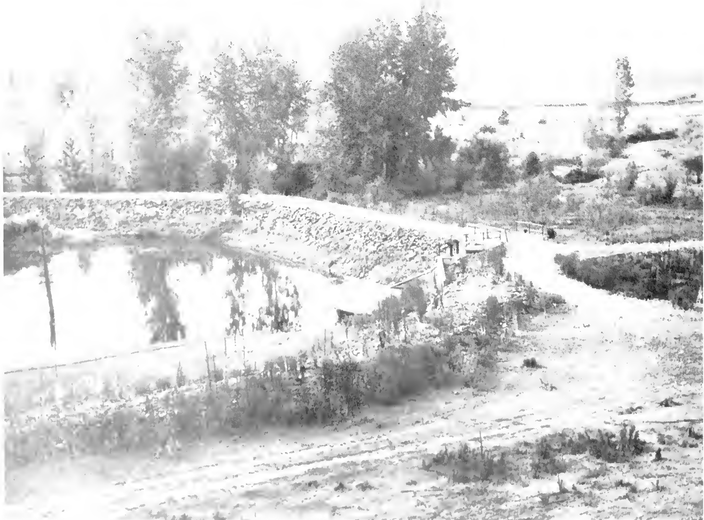
Frenchtown Diversion Dam
