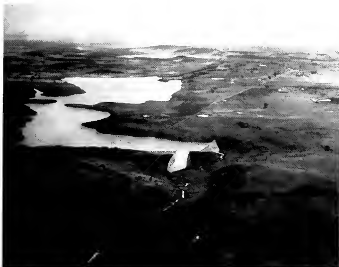
Dawson Draw Dam and Reservoir
