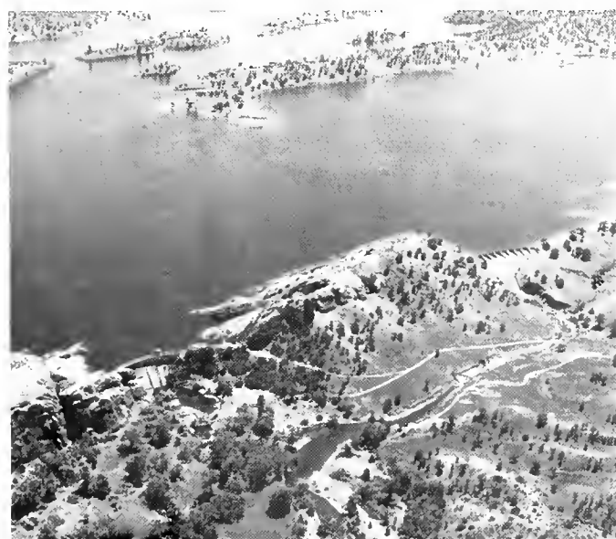
East Park Dam and Reservoir
