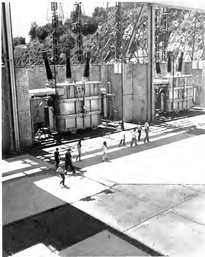
Folsom Dam and Powerplant
