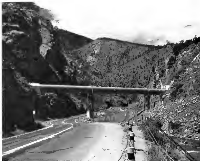
Big Thompson Siphon
