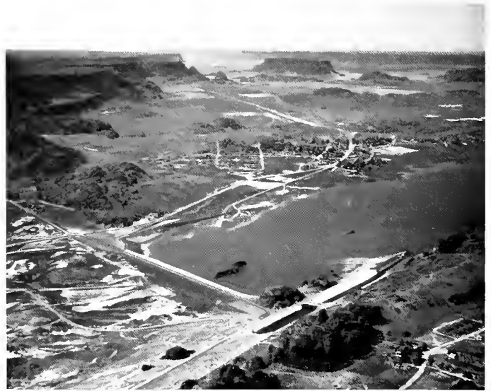
North Dam, Feeder Canal outlet, and Coulee Equalizing Reservoir
