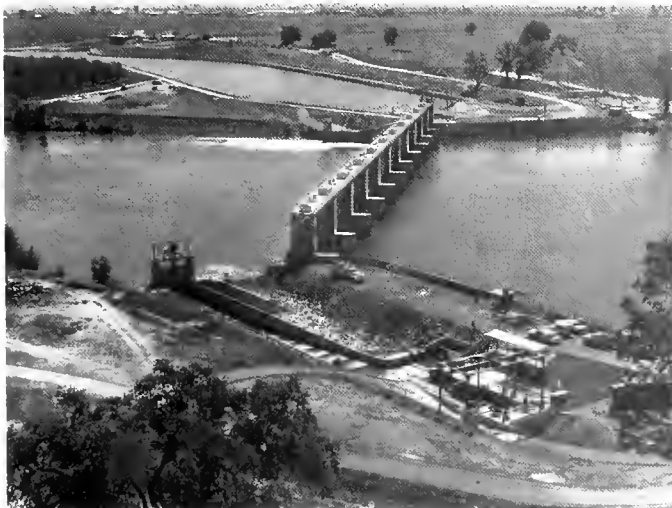
Red Bluff Diversion Dam
