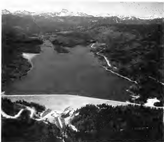
Meeks Cabin Dam and Reservoir
