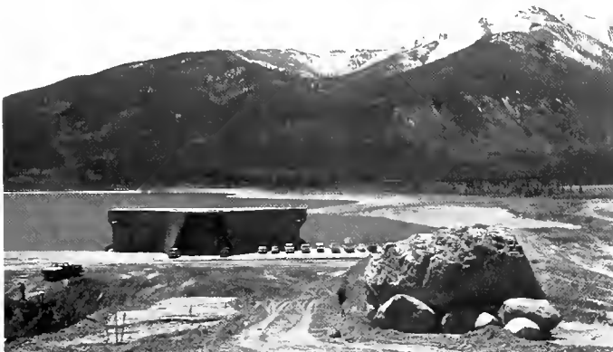
Mt. Elbert Forebay Dam and Reservoir
