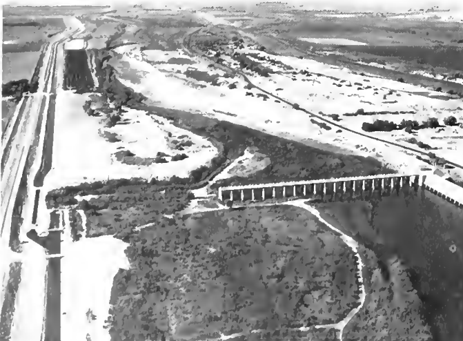
Morelos Dam - U.S. Bypass Drain
