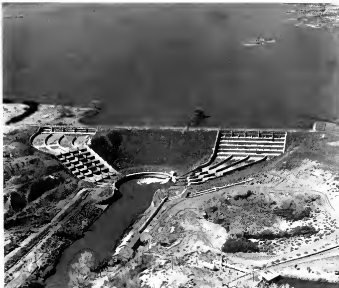
Lahontan Dam and Reservoir
