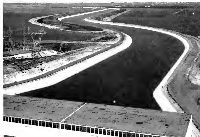
Dos Amigos Pumping Plant and Switchyard
