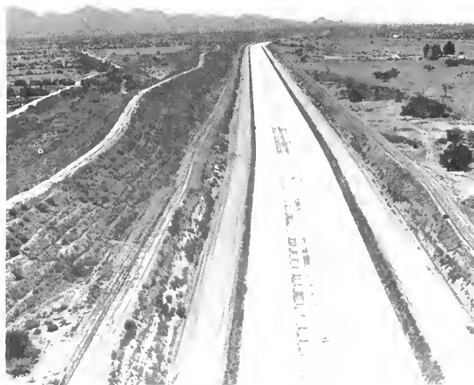
Granite Reef Aqueduct
