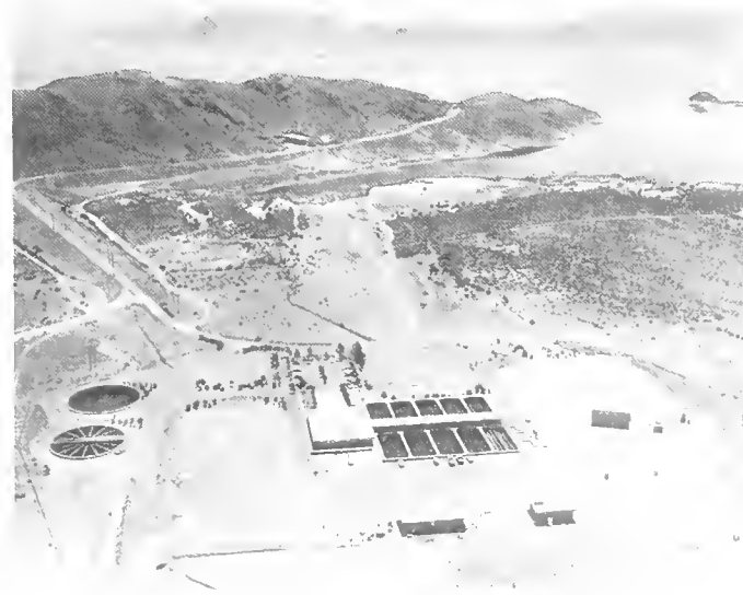
Southern Nevada Water Project Facilities
