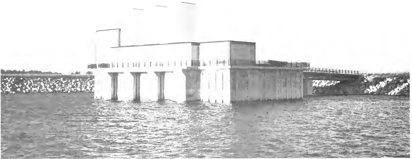
Snake Creek Pumping Plant
