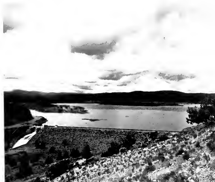
Unity Dam and Reservoir
