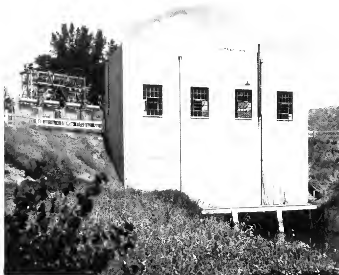
Glendive Pumping Plant
