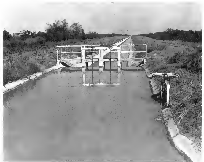
Rehabilitated "F" Lateral
