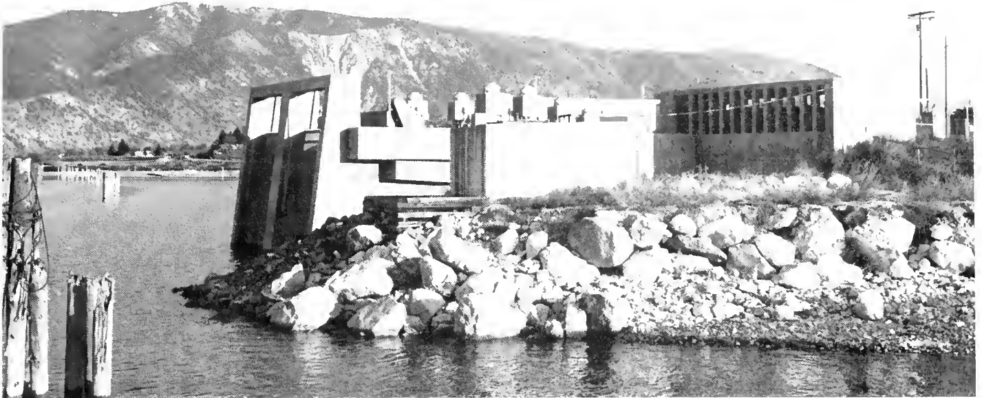
Lake Chelan Pumping Plant
