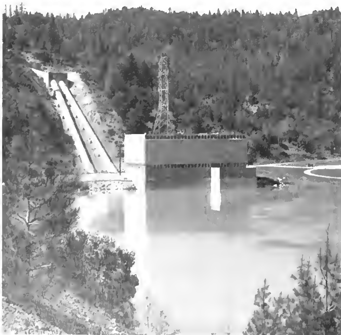
Judge Francis Carr Powerhouse
