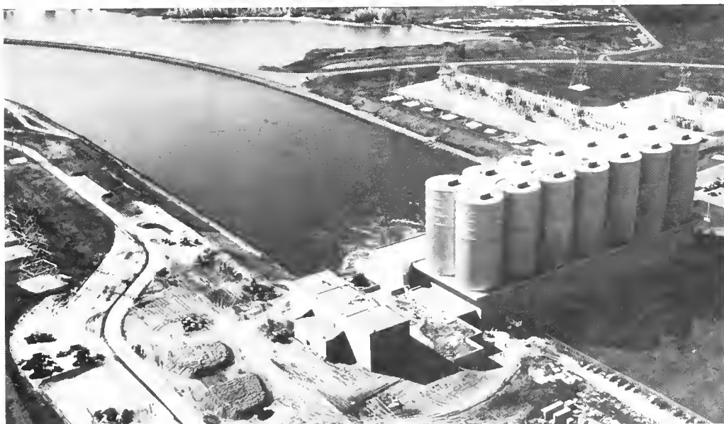
Oahe Pumping Plant
