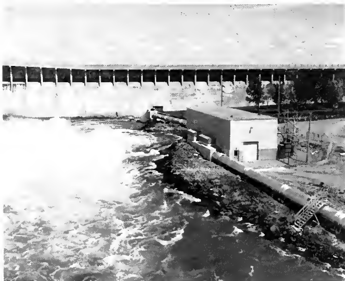
American Falls Pumping Plant
