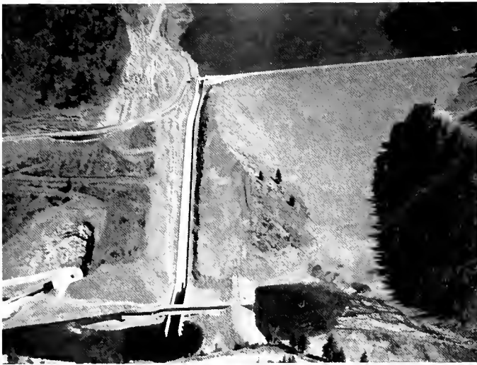
Ruedi Dam and Reservoir
