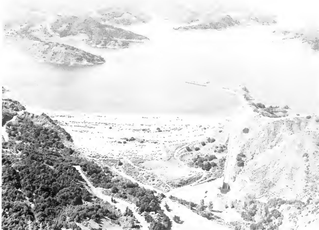
Casitas Dam and Reservoir
