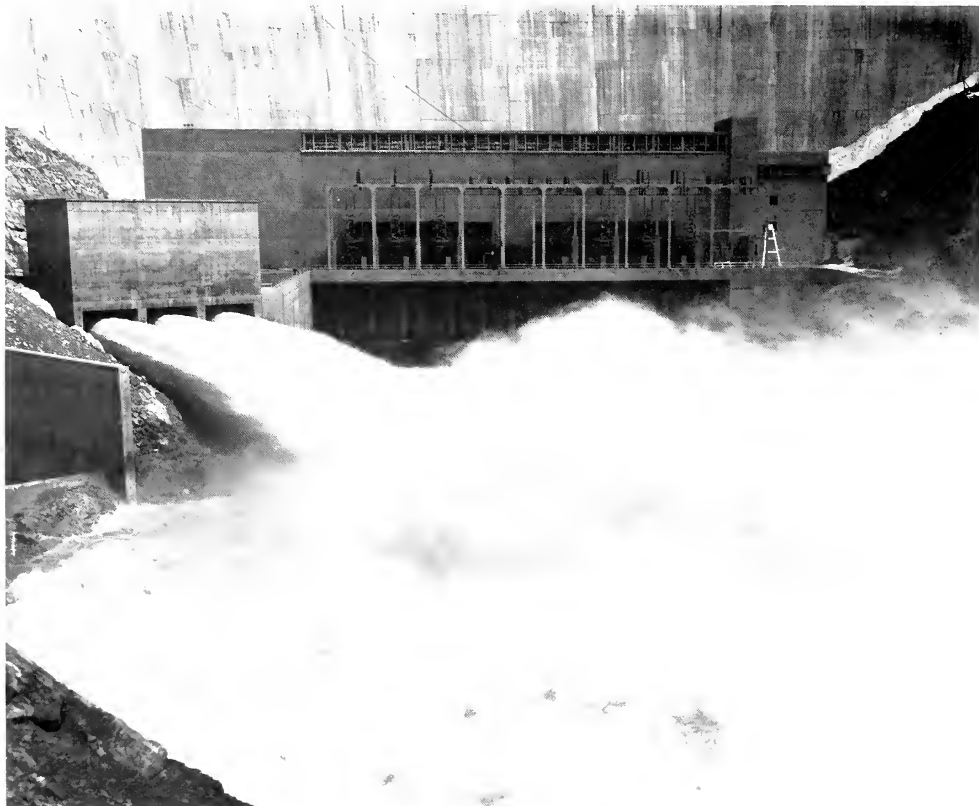
Hollow-jet valve outlets at Hungry Horse Dam
