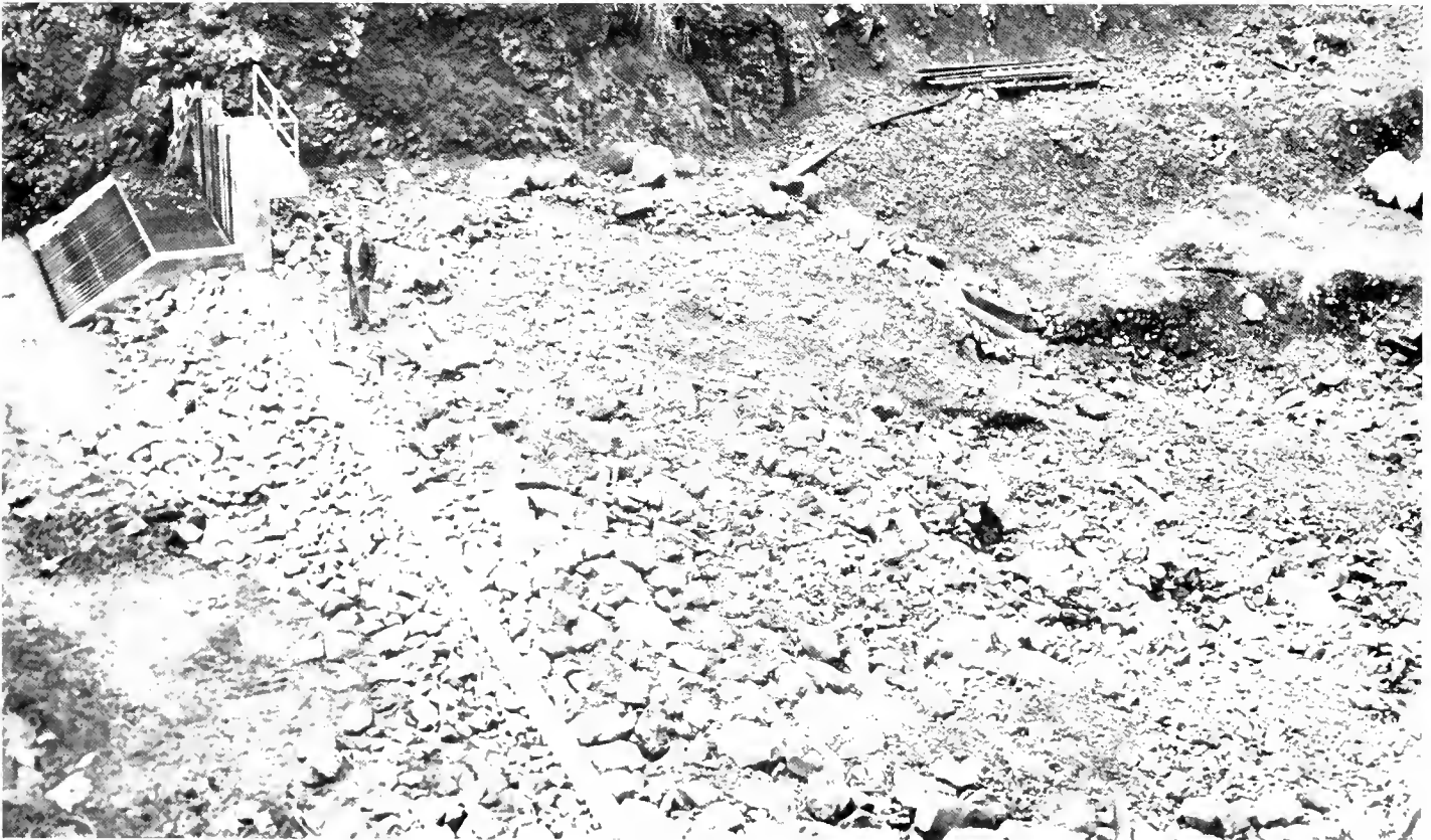
Webb Creek Diversion Dam
