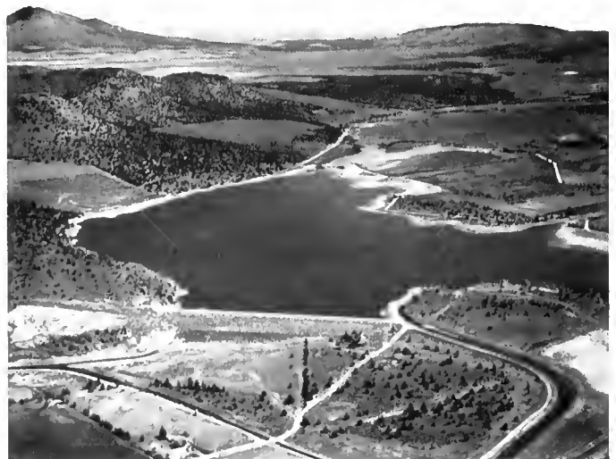
Haystack Dam and Reservoir
