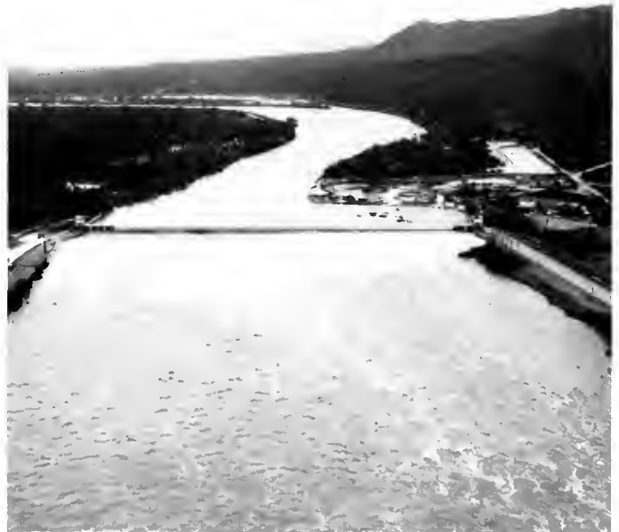
Granite Reef Diversion Dam
