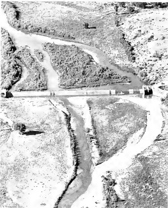
Fort Sumner Diversion Dam
