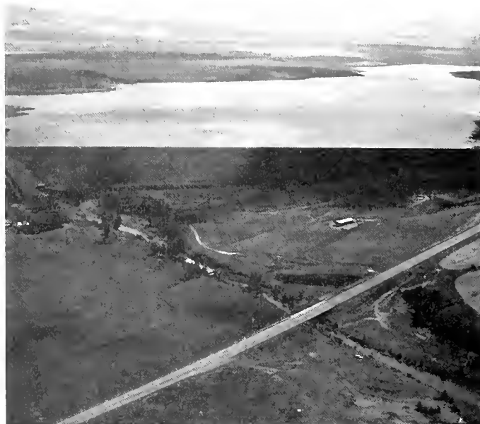
McKay Dam and Reservoir
