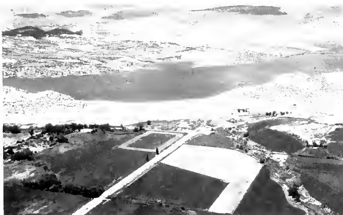
Steinaker Dam and Reservoir
