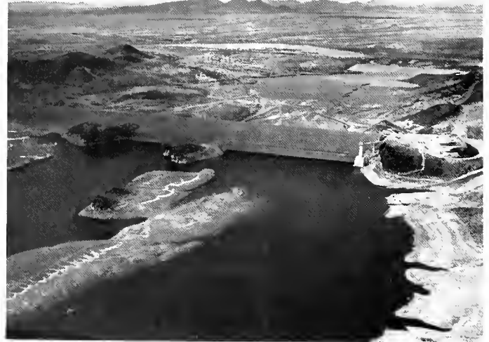
Painted Rock Dam and Reservoir
