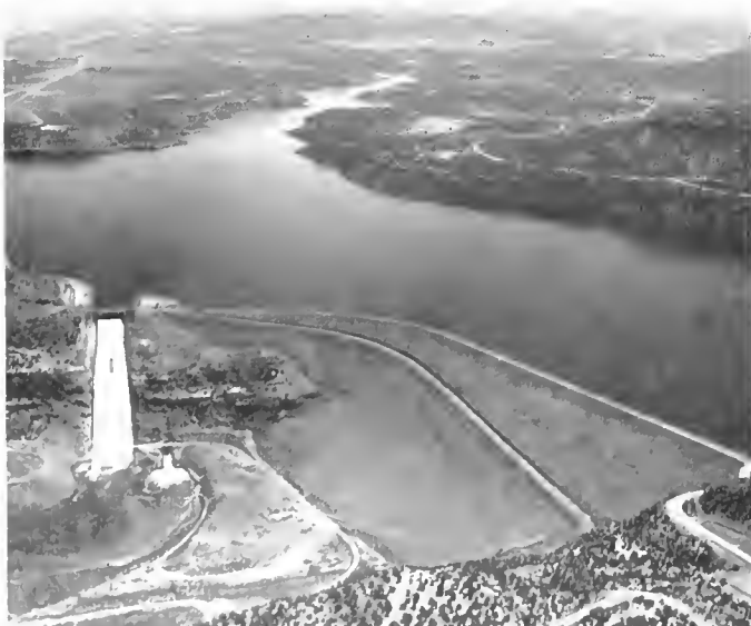
Navajo Dam and Reservoir
