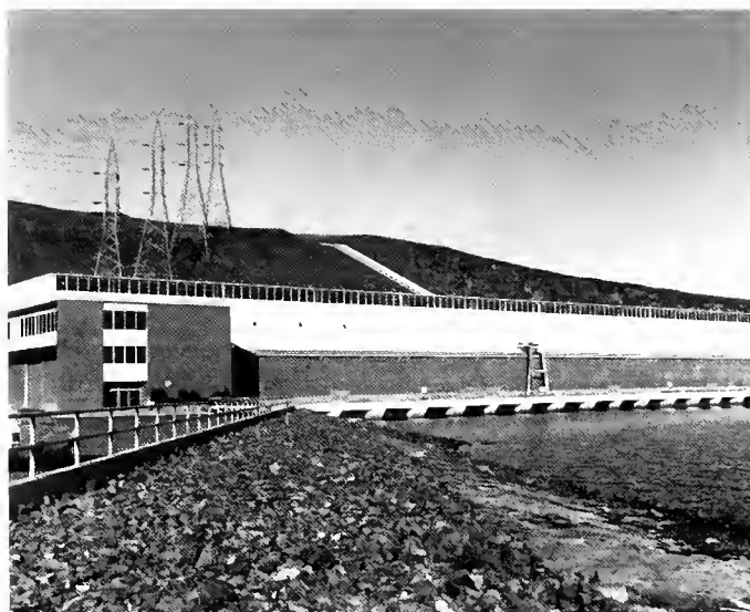
San Luis Pumping-Generating Plant
