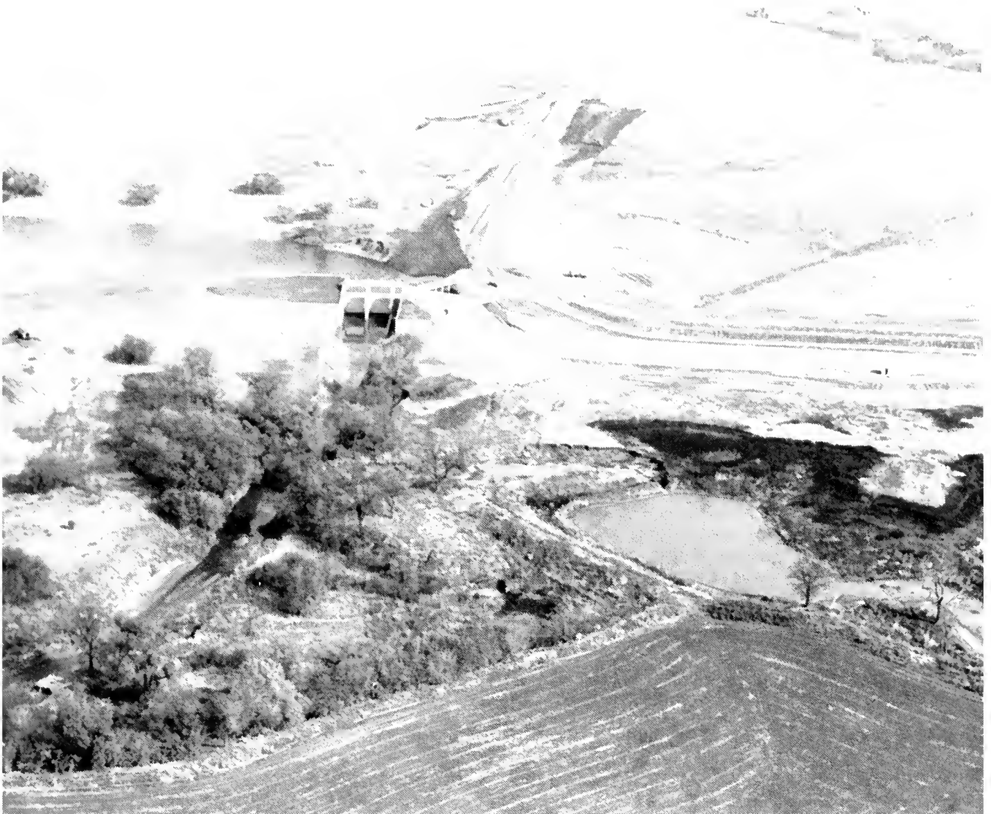
Bretch Diversion Dam and Canal
