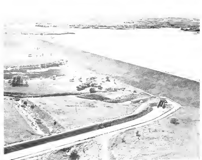
Sherman Dam and Reservoir
