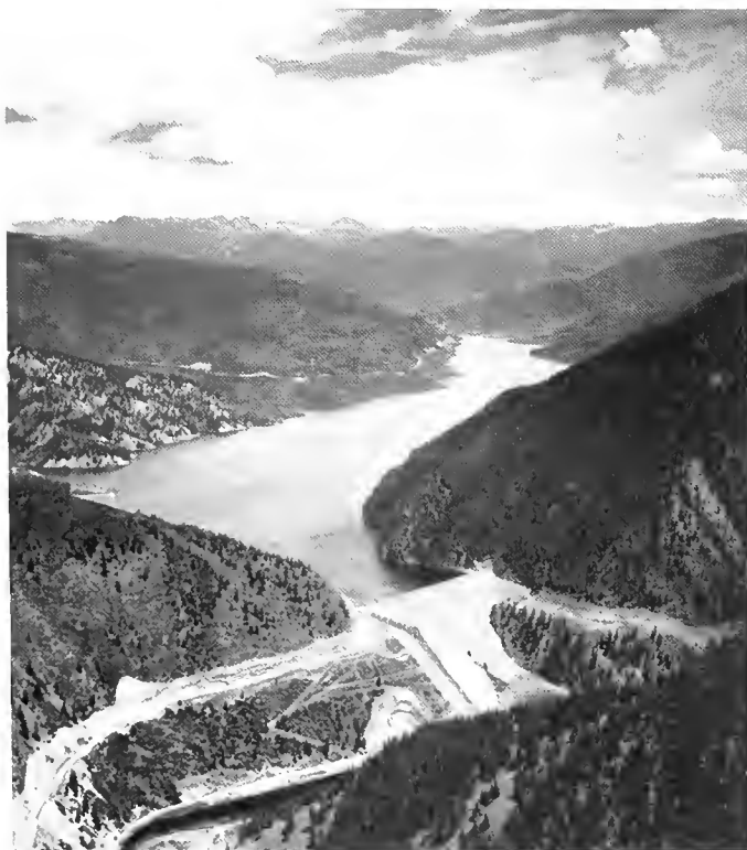
Ruedi Dam and Reservoir
