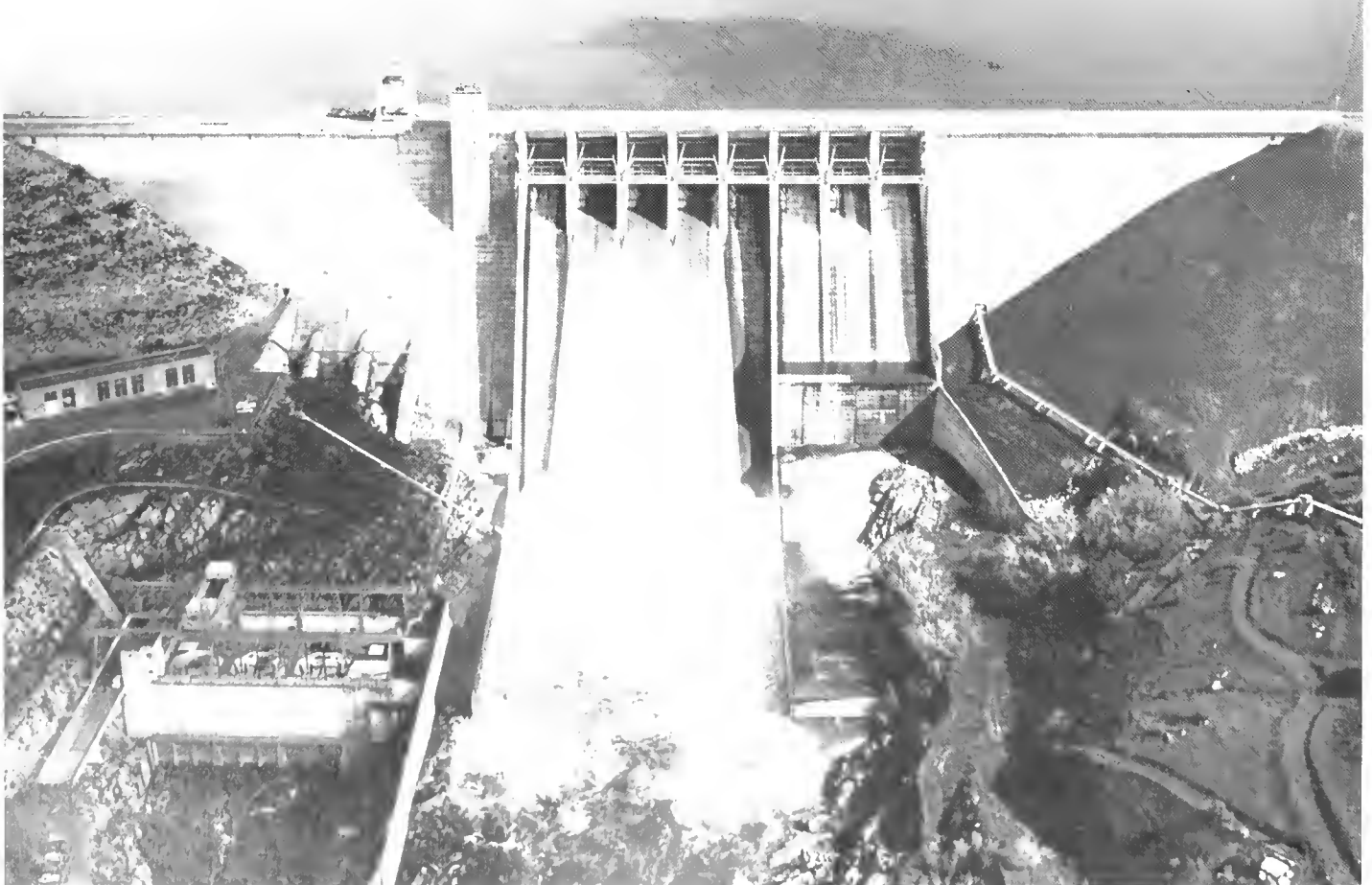
Folsom Dam, Powerplant, and Lake
