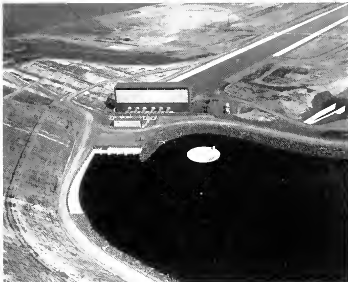
O'Neill Forebay Pumping Plant
