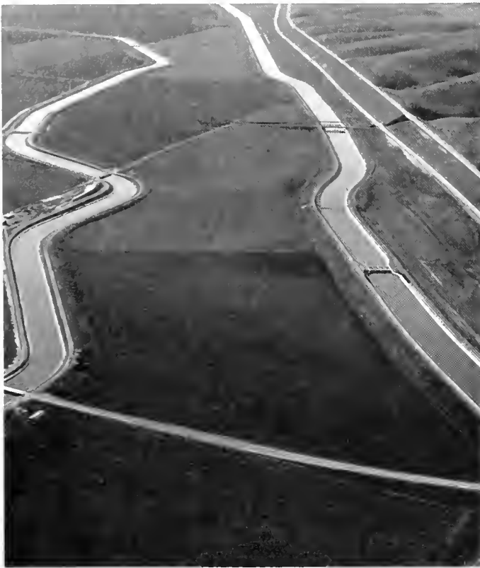
Delta-Mendota Canal and California Aqueduct
