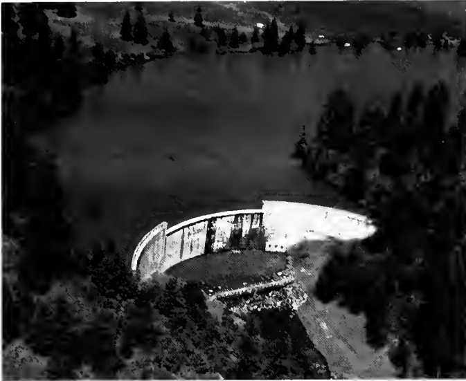
Gerber Dam and Reservoir
