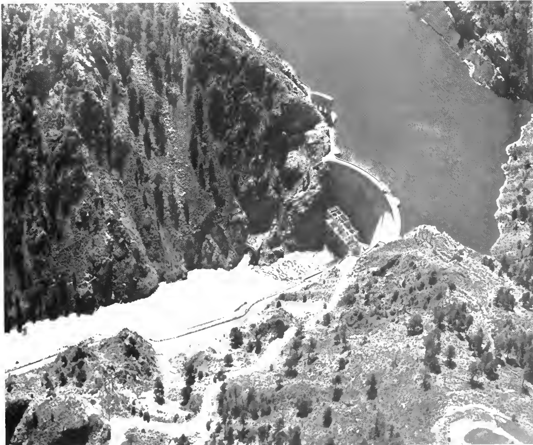
Seminoe Dam and Powerplant
