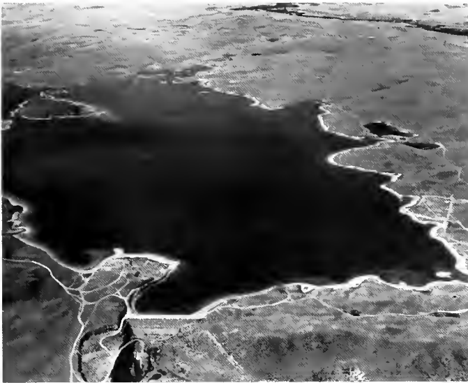
Willow Creek Dam and Reservoir
