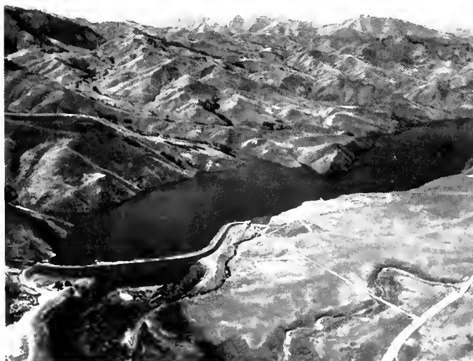
Little Wood River Dam and Reservoir
