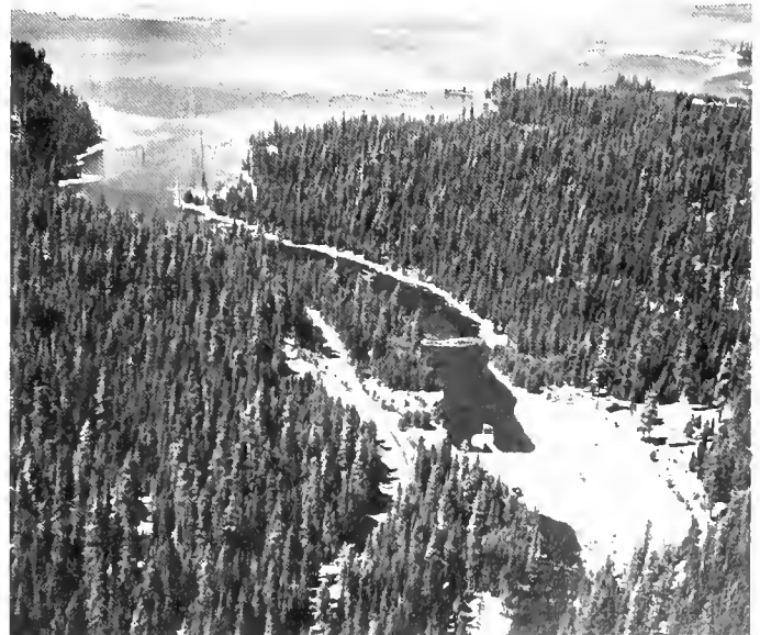
Crane Prairie Dam
