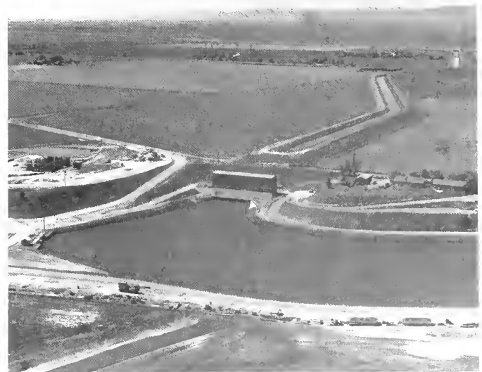
Corning Pumping Plant
