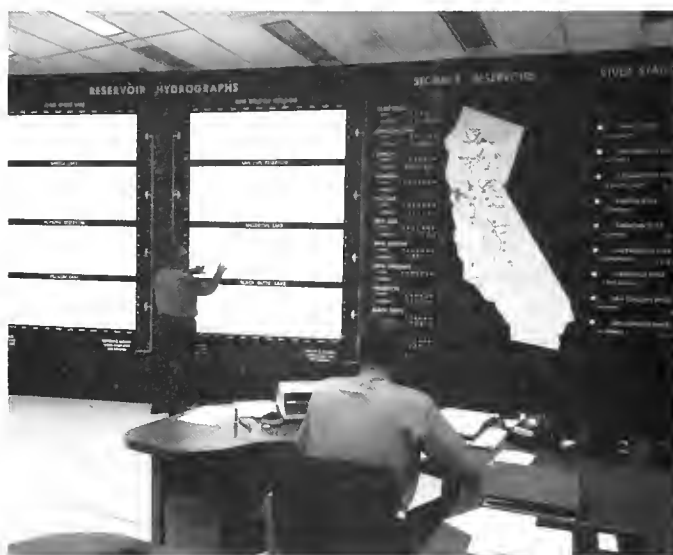
Central Valley Operations Control Center
