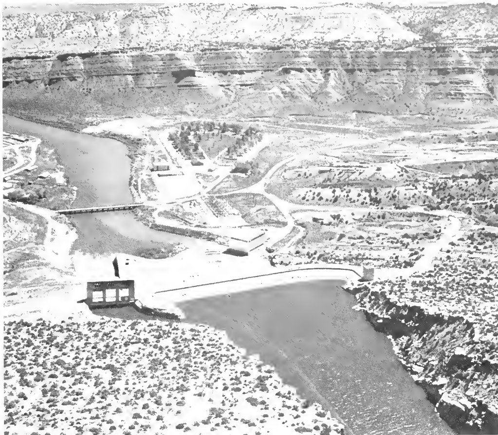
Alcova Dam and Powerplant
