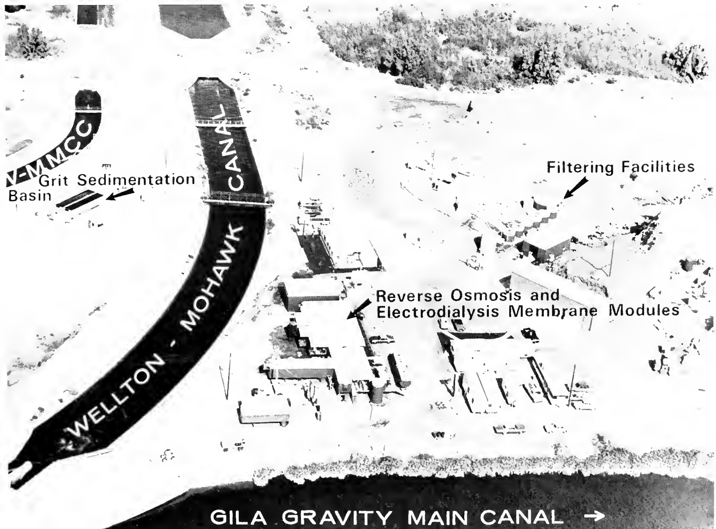
Yuma Desalting Test Facility
