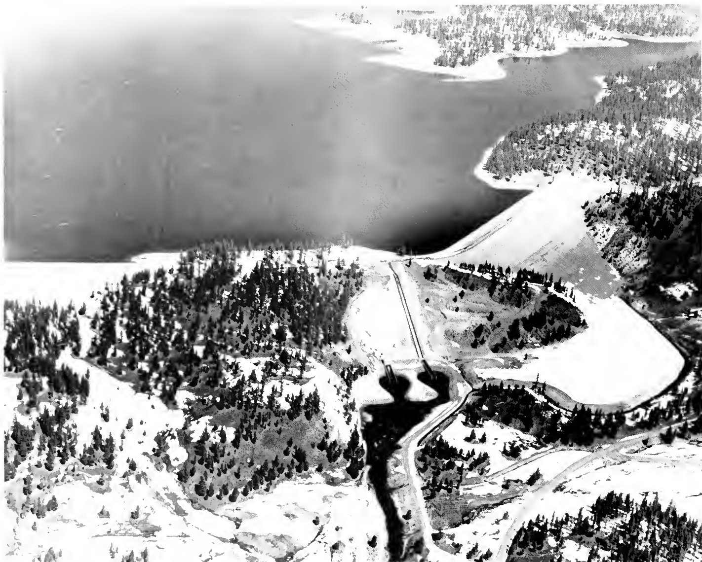
Stampede Dam and Reservoir
