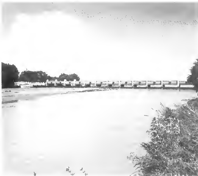
Mesilla Diversion Dam
