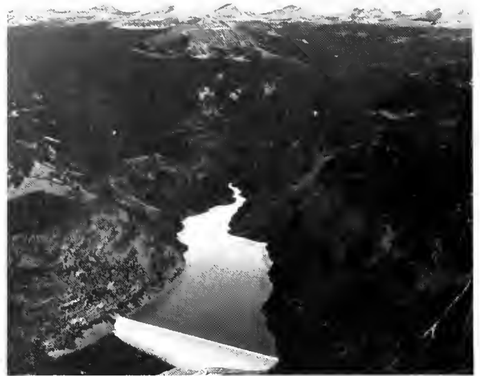
Upper Stillwater Dam and Reservoir
