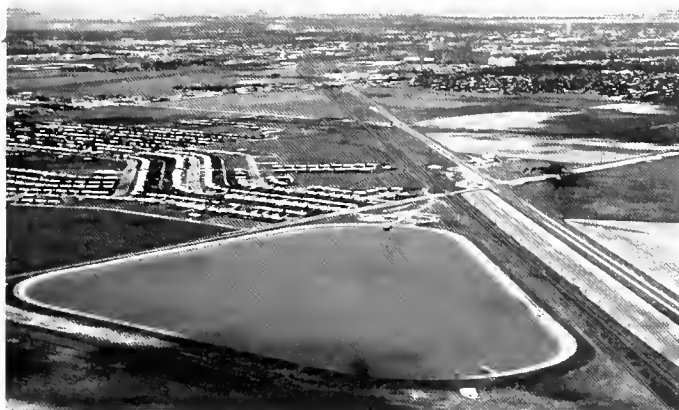
Amarillo Regulating Reservoir
