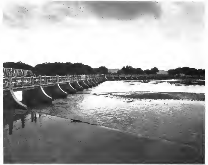
Isleta Diversion Dam
