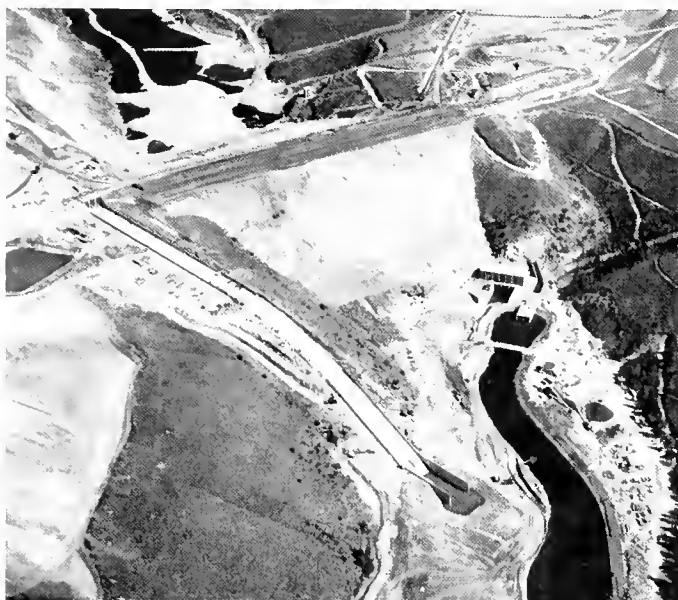
Teton Dam before failure
