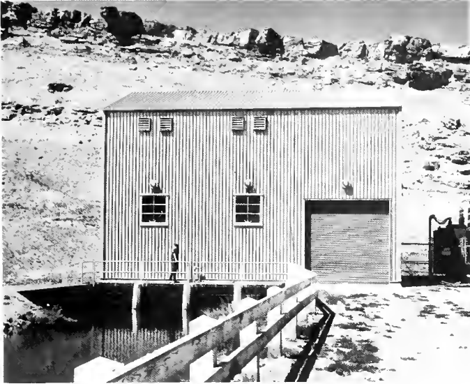
Lucerne Pumping Plant No. 1
