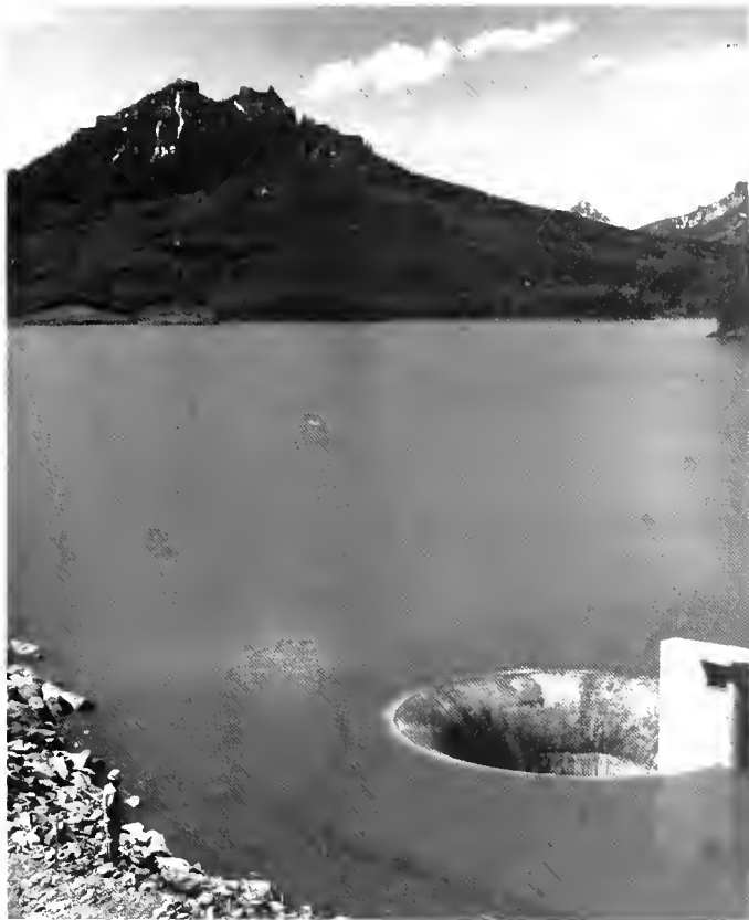
Morning-glory spillway intake structure
