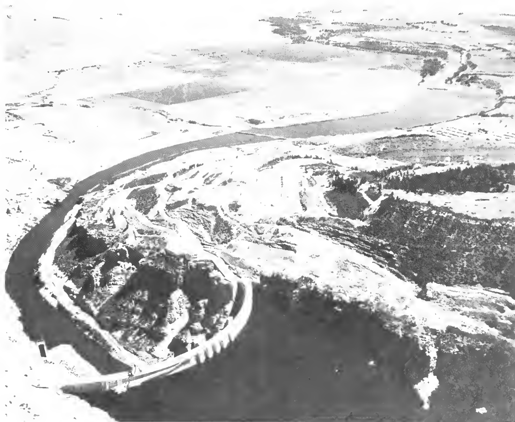
Yellowtail Dam and Afterbay Dam
