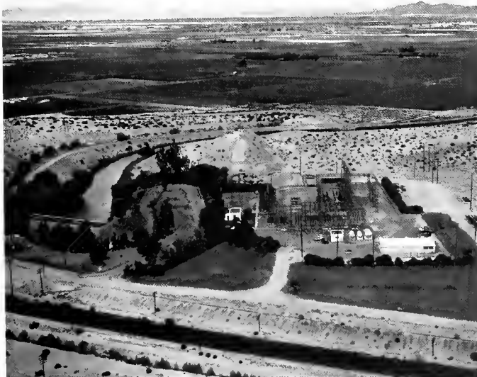
Yuma Mesa Pumping Plant and Gila Substation
