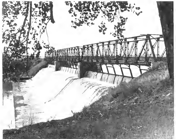
Dodson Diversion Dam
