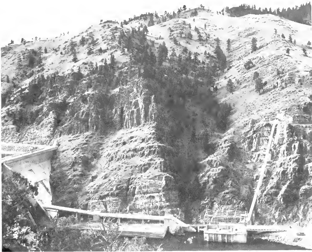
Helena Valley Pumping Plant
