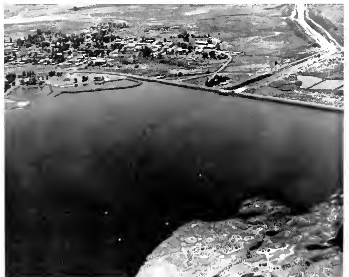
Banks Lake, Dry Falls Dam, outlet works, and Main Canal
