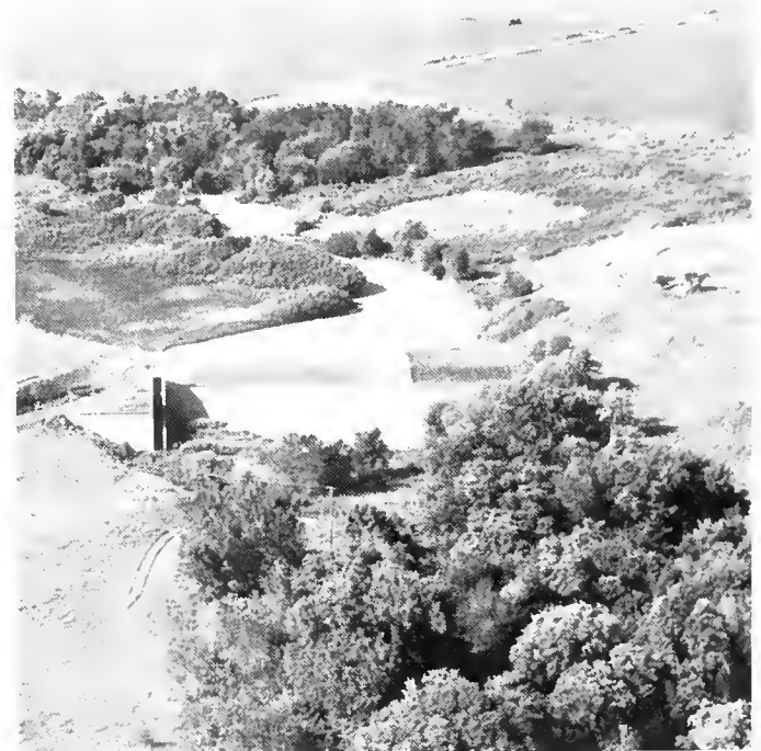
Almena Diversion Dam
