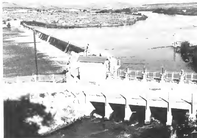
Leasburg Diversion Dam
