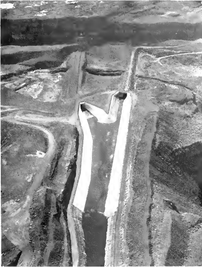
Inlet of Bacon Siphon and Tunnel
