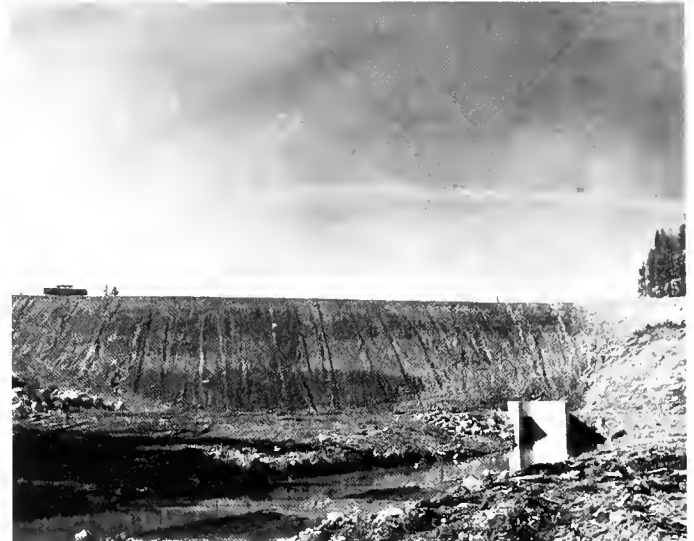
Outlet works stilling basin at Wasco Dam
