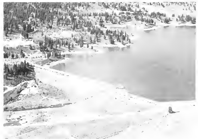
Boca Dam and Reservoir
