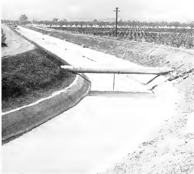
Putah South Canal
