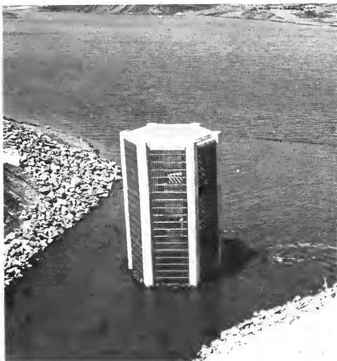
Outlet works intake structure at Stampede Dam
