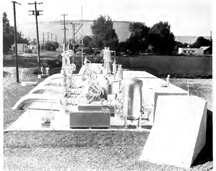
Barnes Butte Pumping Plant
