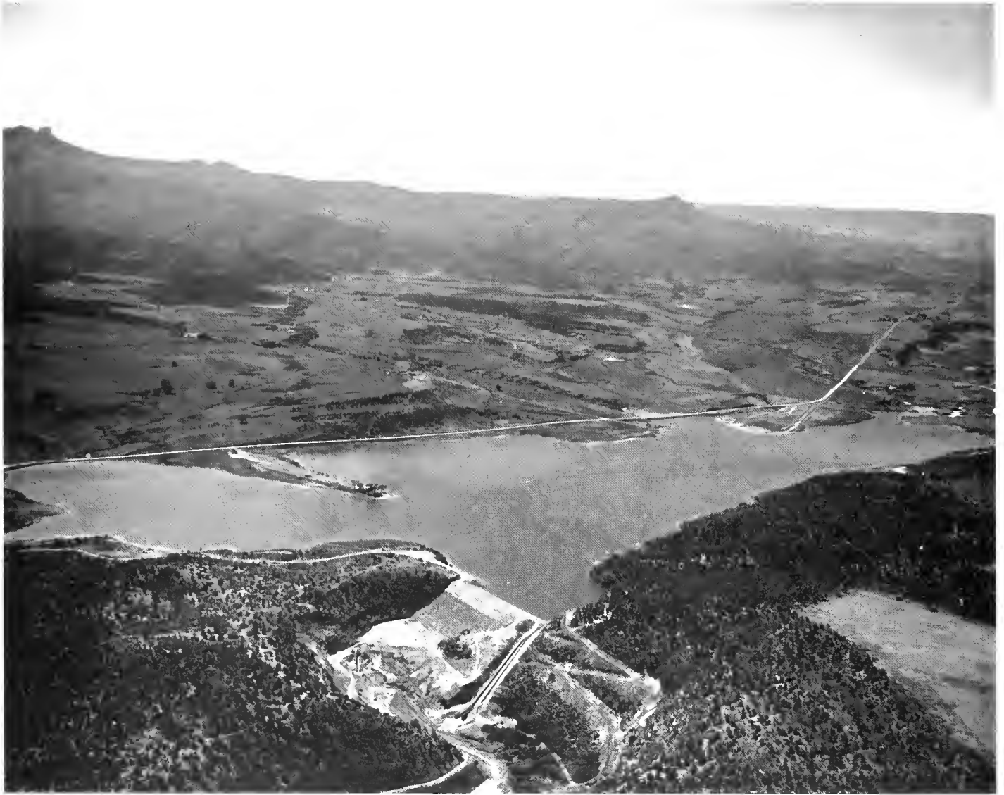
Crawford Dam and Reservoir
