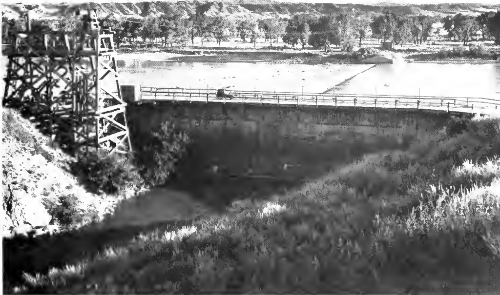
Lower Yellowstone Diversion Dam
