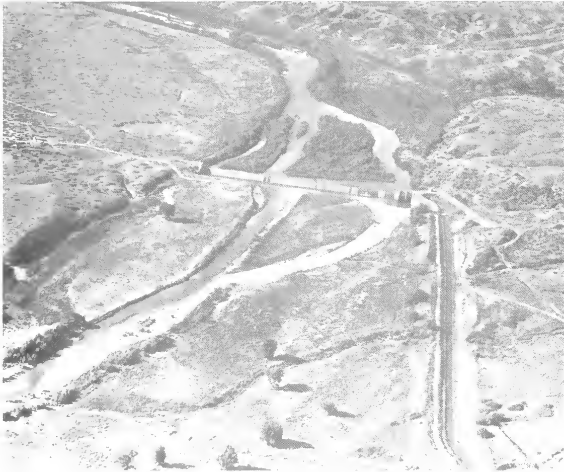
Fort Sumner Diversion Dam
