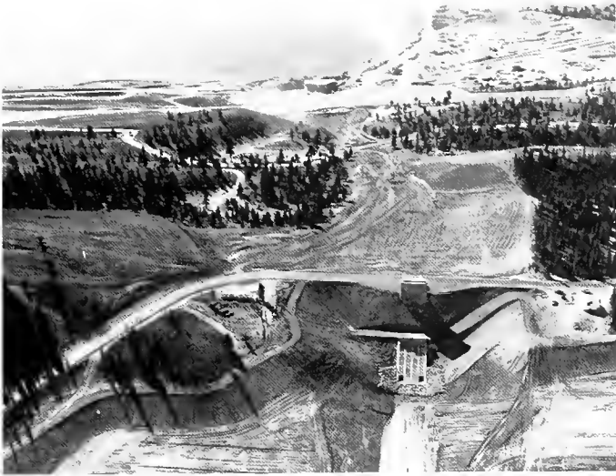
Mt. Elbert Forebay Dam and Reservoir
