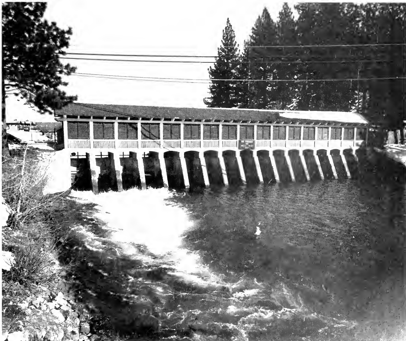
Lake Tahoe Dam
