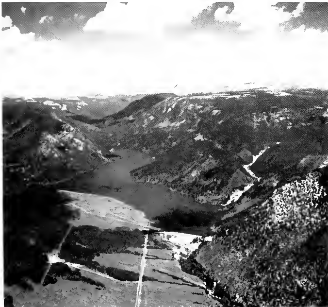
Moon Lake Dam and Reservoir
