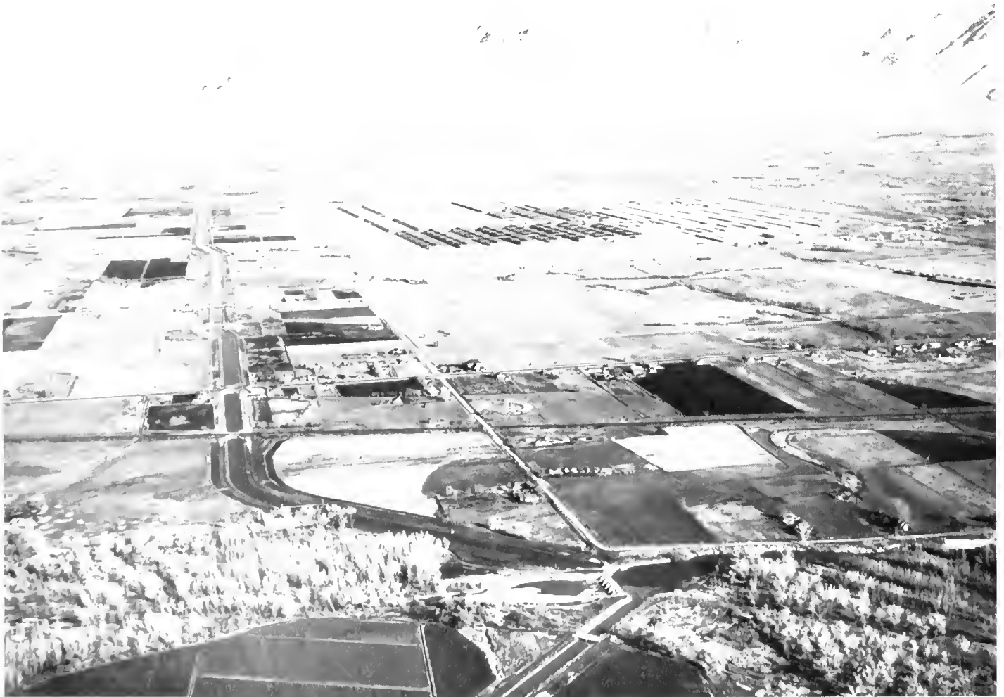
Slaterville Diversion Dam and Willard Canal
