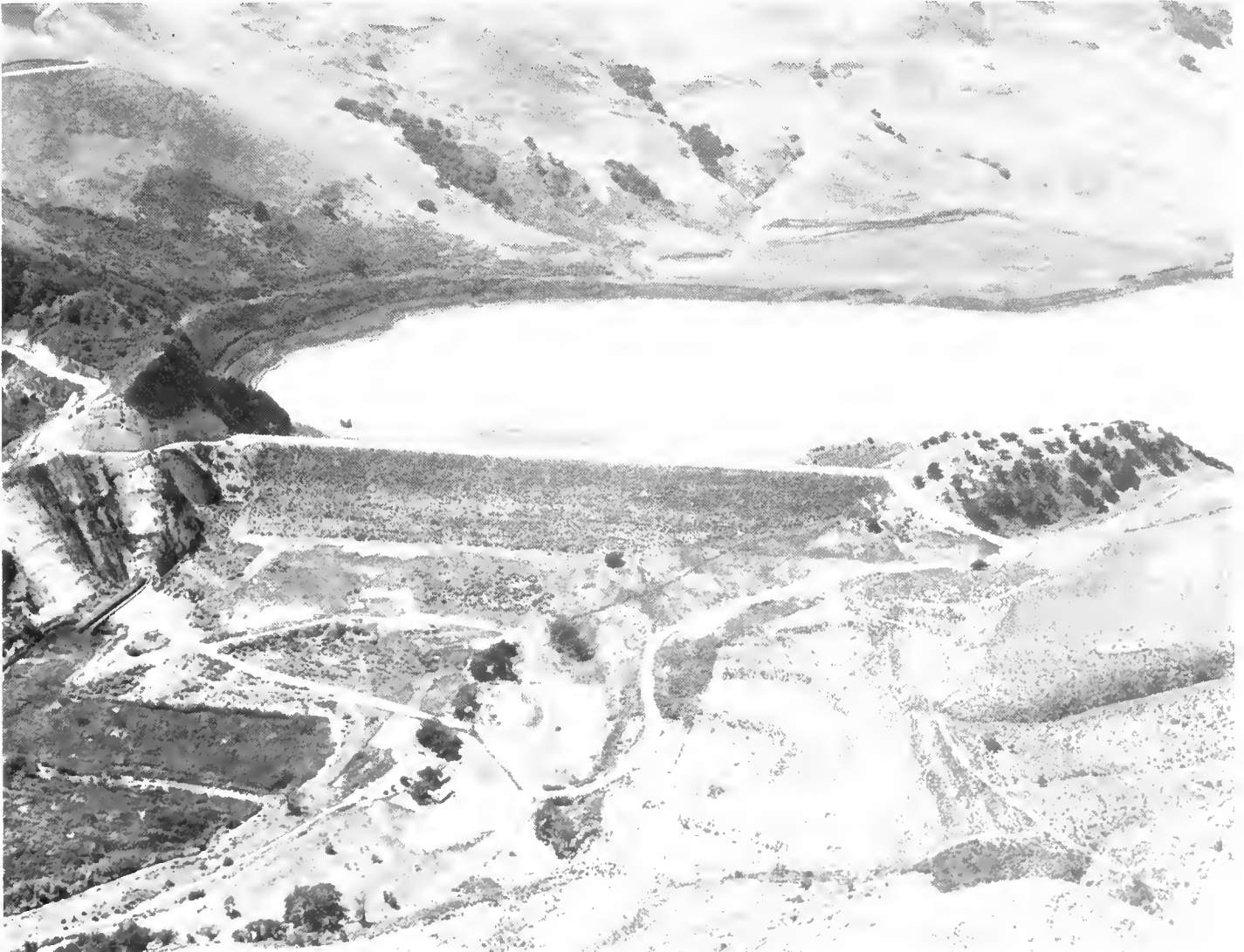
Twitchell Dam and Reservoir
