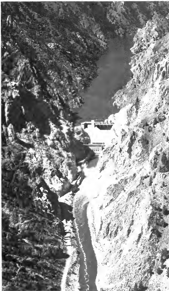
Kortes Dam and Powerplant
