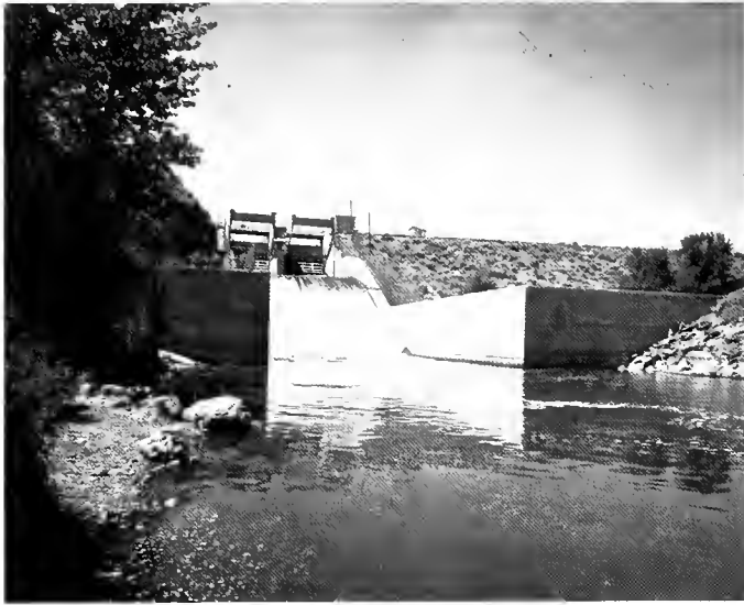
Unity Dam spillway
