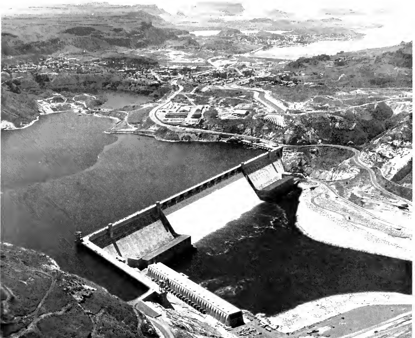
Grand Coulee Dam, Powerplants, and Pumping Plant
