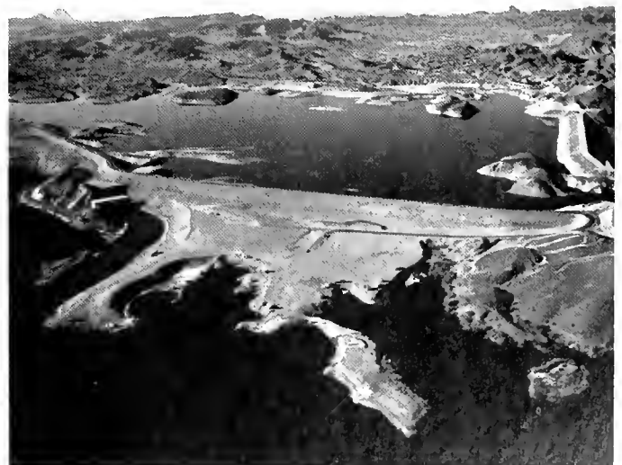
Imperial Dam and Reservoir
