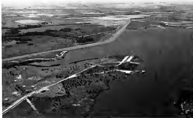
Fort Cobb Dam and Reservoir
