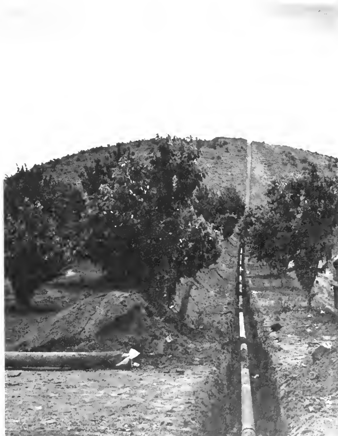
Placing pipe for distribution system
