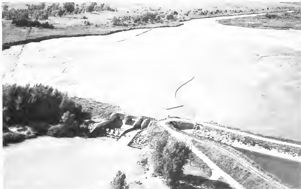
Milburn Diversion Dam
