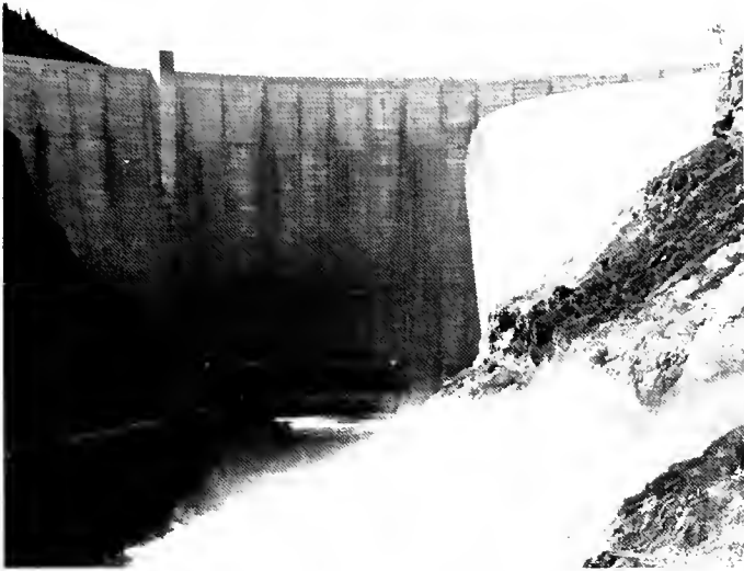
Yellowtail Dam spillway release
