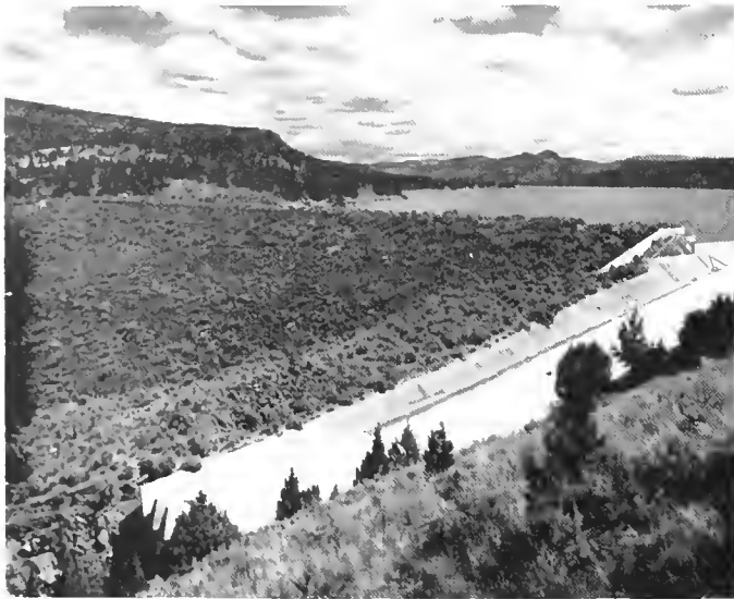
Open, concrete-chute spillway at Ochoco Dam
