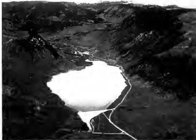
Lower Stillwater Dam and Reservoir
