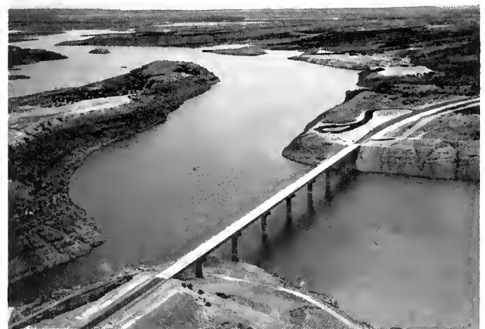
Bridge crossing Starvation Reservoir
