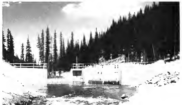
South Fork Diversion, South Side Collection System
