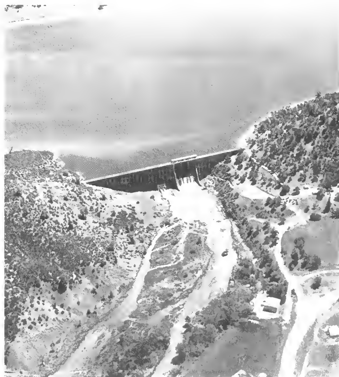
Stony Gorge Dam and Reservoir
