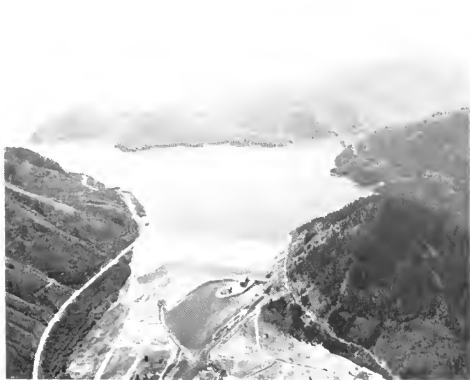
Palisades Dam and Reservoir
