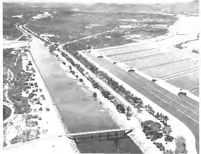
Laguna Settling Basin, All-American Canal Desilting Basin, and All-American Canal
