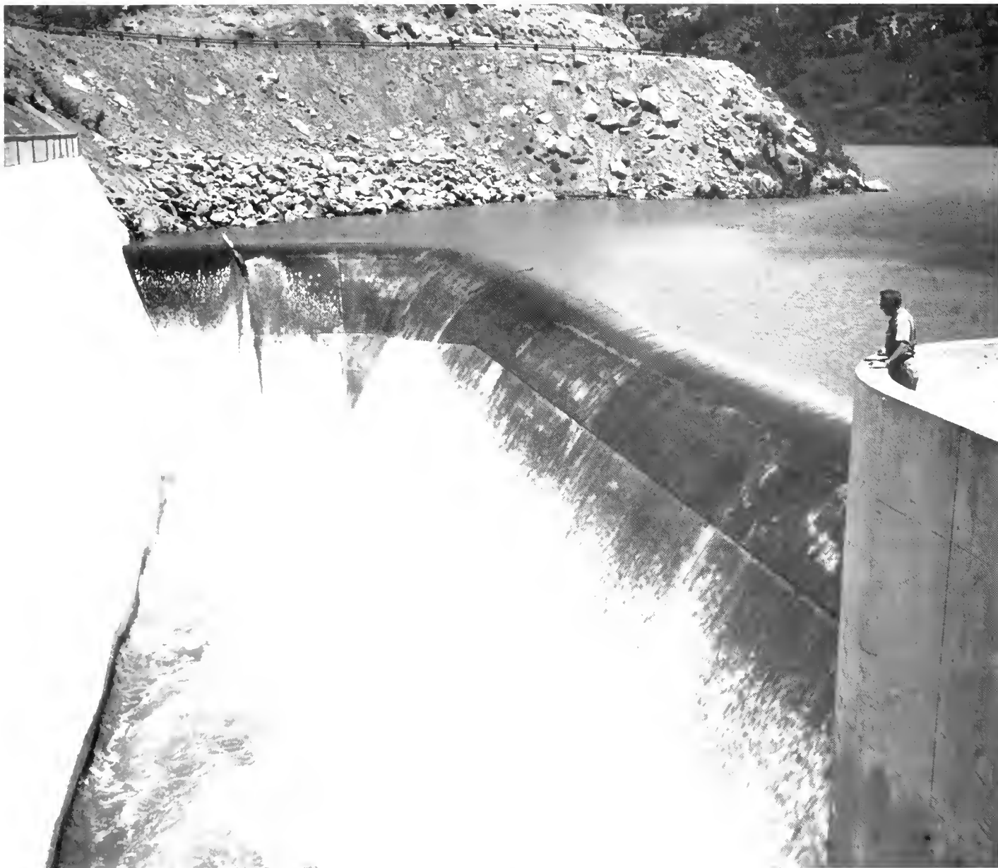
Spillway inlet structure
