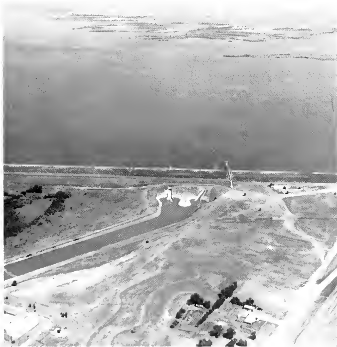
Cheney Dam and Reservoir
