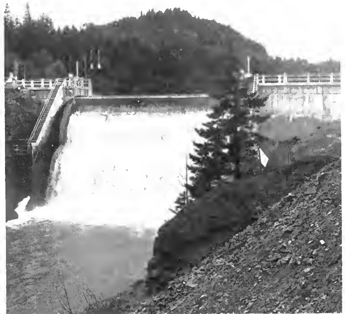
Easton Diversion Dam
