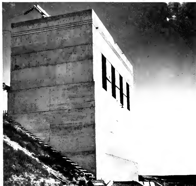
Shirley Pumping Plant
