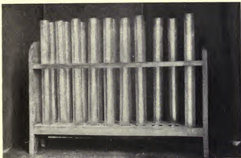
FIG. 61.—Color Standards and Rack.
