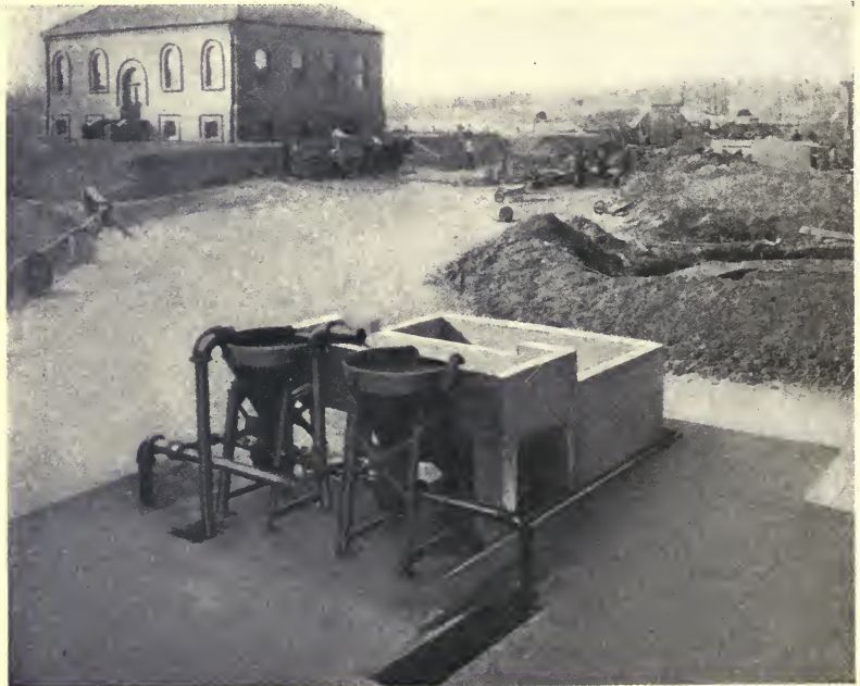
FIG. 23.—Sand Washers, Washington Filtration Plant.
