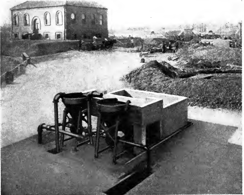
FIG. 23.—Sand Washers, Washington Filtration Plant.
