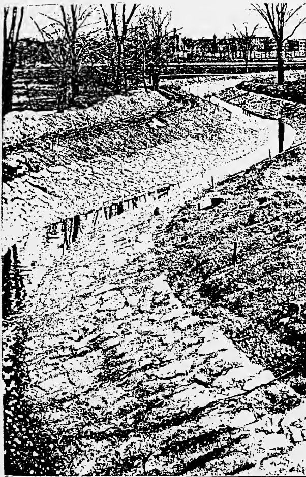
IMPROVEMENT OF CANTERBURY BRANCH OF STONY BROOK.
