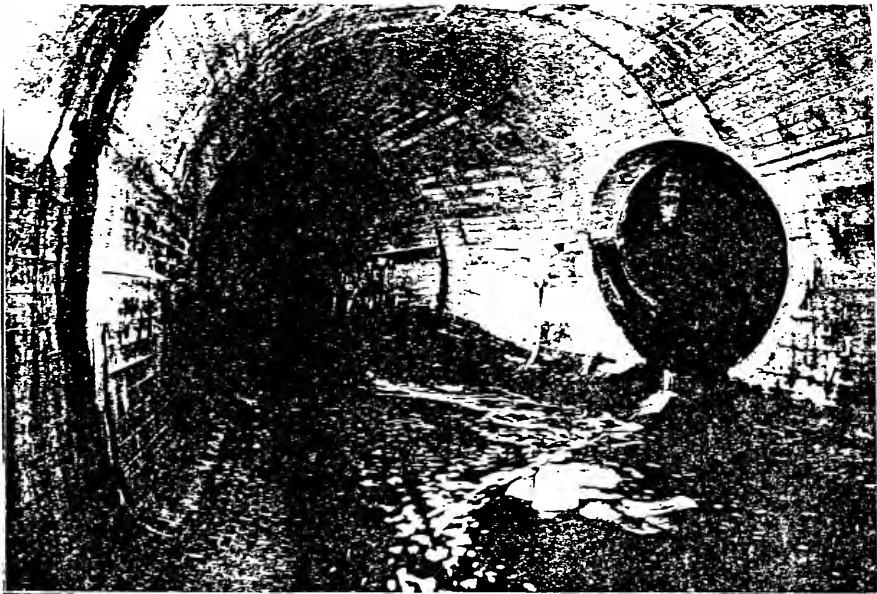
JUNCTION MAIN CHANNEL STONY BROOK AND BUSSEY BROOK BRANCH CONDUIT AT REDUCER ON MAIN CHANNEL AT FOREST HILLS SQUARE.
