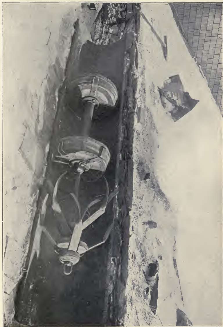
Fig. 94.—Pipe-SCRAPER.
