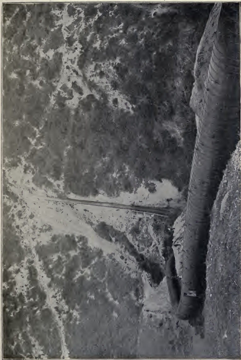
PLATE XI.—WOODEN-STAVE PIPE. (From Trans. Am. Soc. C. E., Vol. XXXIII.)
