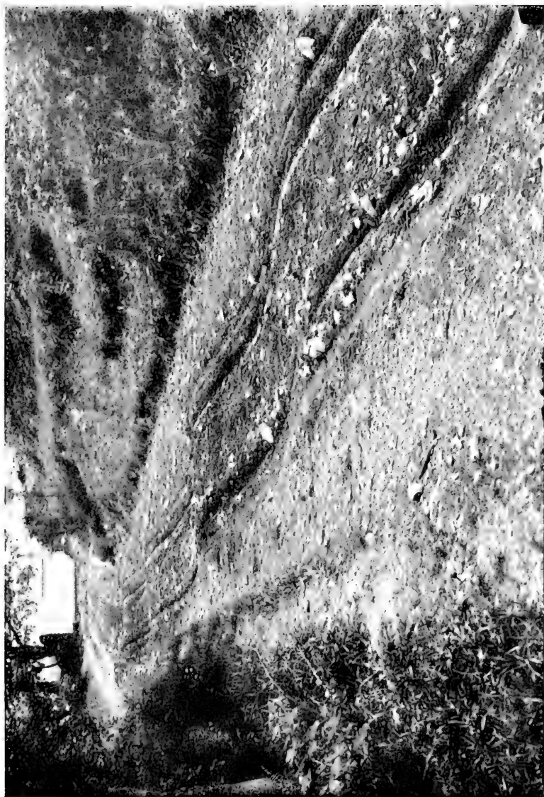
PLATE 47.—“Cahots,” the undulations made in a road by the sledges which descend from the Saddlestone Quarry, Coniston, Lancs.
