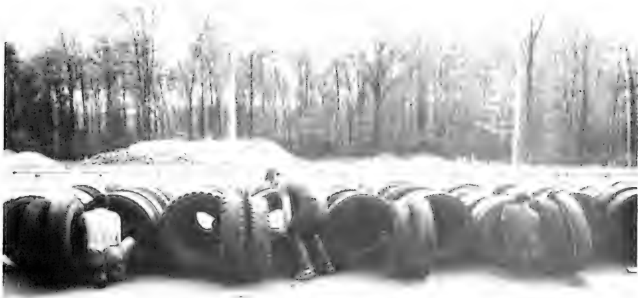
Figure 14. Belts are overlapped and bolted together.
