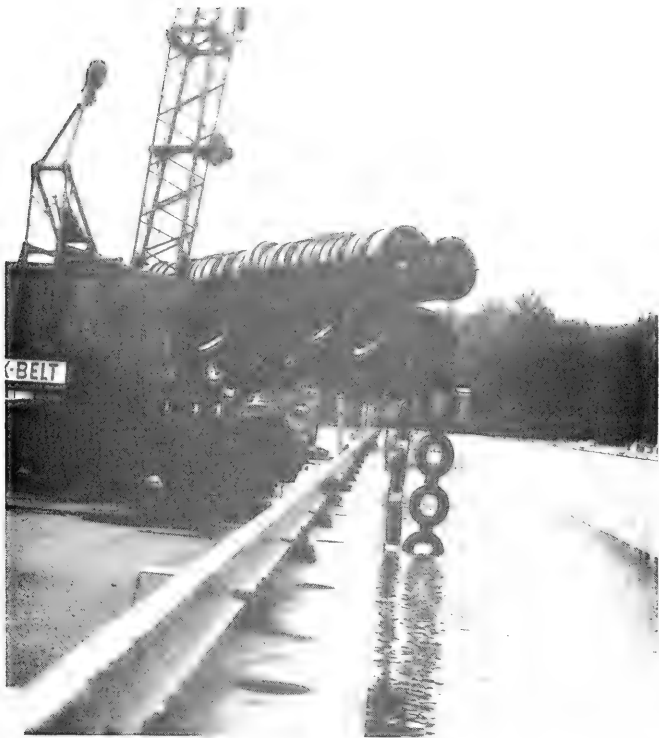
Figure 21. Inserting PT-1 breakwater.
