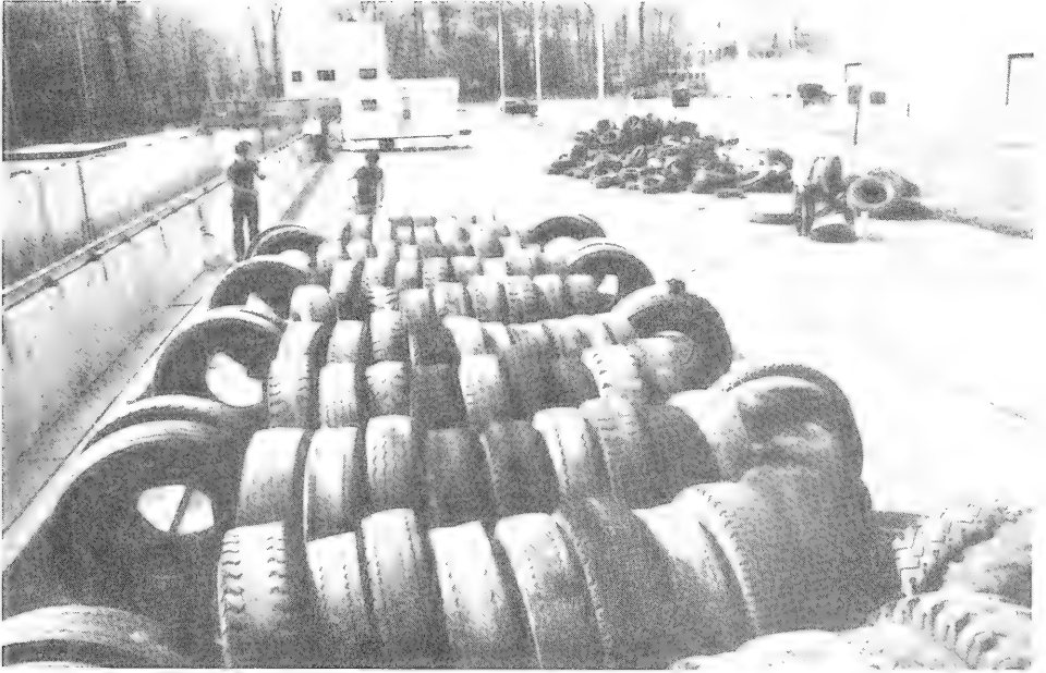
Figure 11. Tires are in position, ready to be tied.
