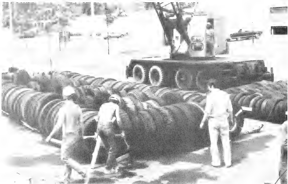
Figure 16. PT-1 module ready for lift into wave tank.
