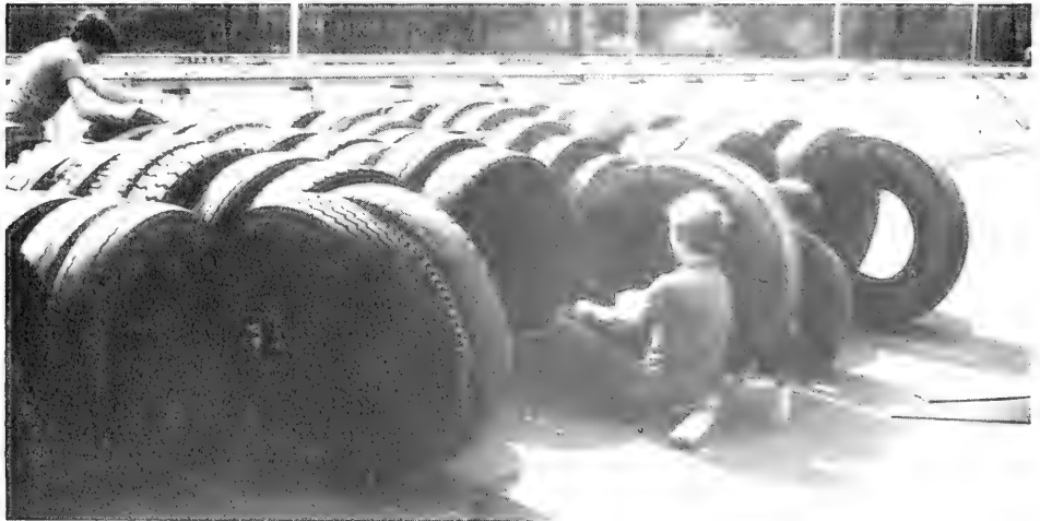
Figure 13. Tensioning belt before completing belt-to-belt connection.
