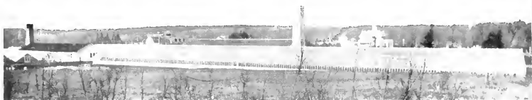
Iron Frame Carnation House, 30x300, erected by the Lord & Burnham Co. for the Chicago Carnation Co., Joliet, Ill., last summer.
