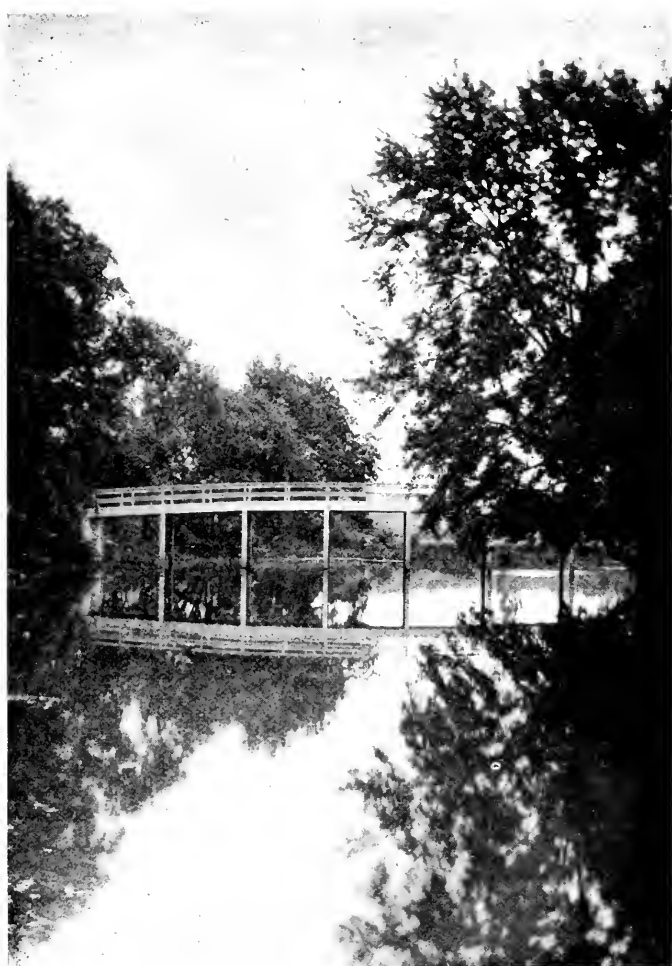
The bridge at the Battleground
