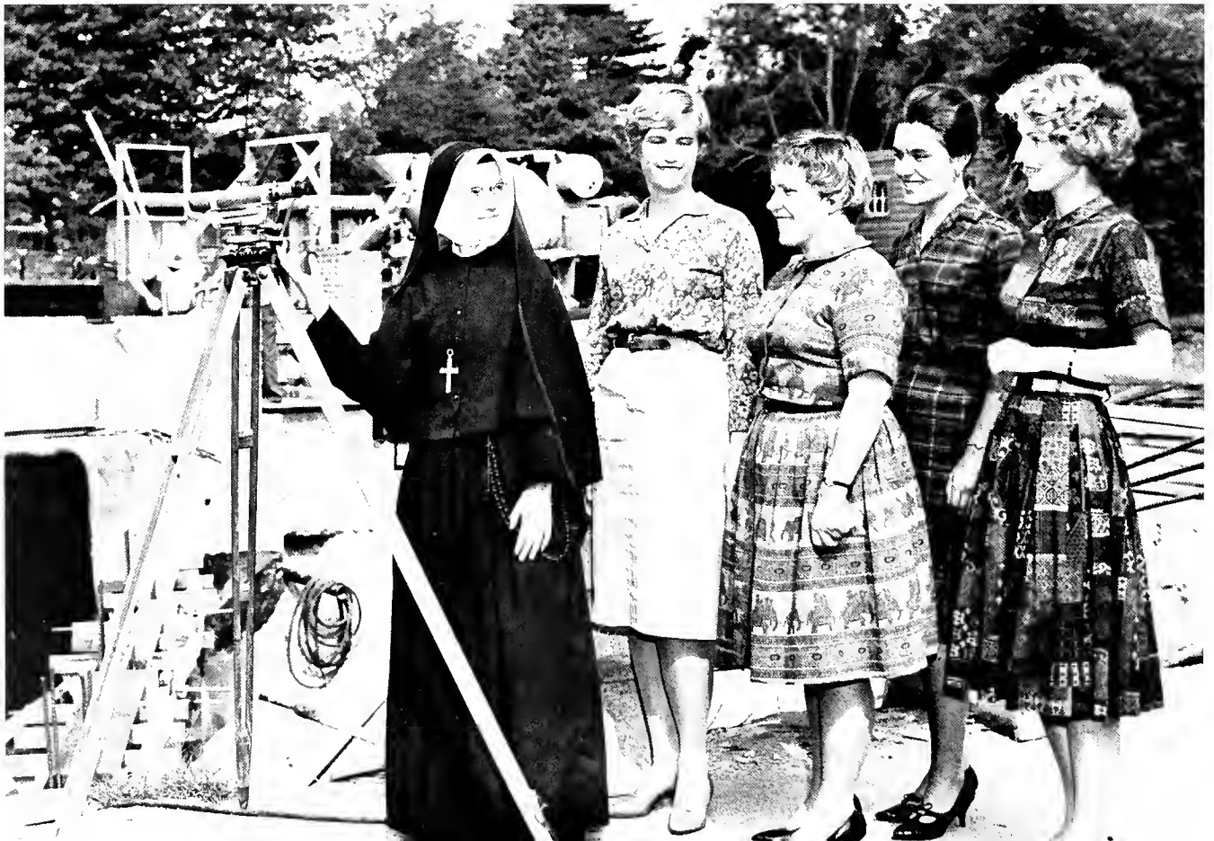
Toward the concrete
