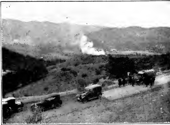
THE STATE GOVERNMENT BUILDS ROADS. This interesting photograph shows where a road built by one state stops at the boundary line of its neighboring state. A state government BUILDS
