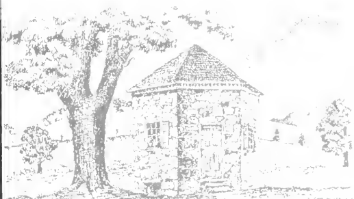
The Hexagonal Schoolhouse c. 1837, Cambria Township, Pennsylvania
