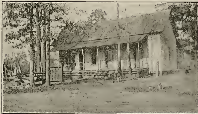
Another little cabin. There are perhaps fifty or sixty of about this type. New temporary houses are now being built.
