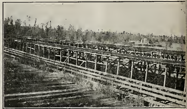
These high plank walks contain hundreds of thousands of feet of lumber, much of it still good for building purposes.
