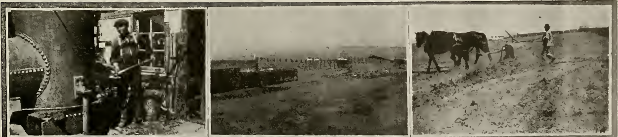
Left, firing boiler at south industrial building; center, stone work for horse barn; right, grading Llano land for irrigating.
