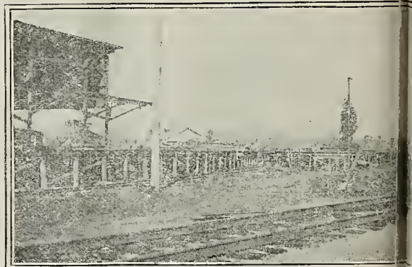
The Left Shows the North-West Corner of the Warehouse. In Foreground is the Kansas City Southern Railroad
