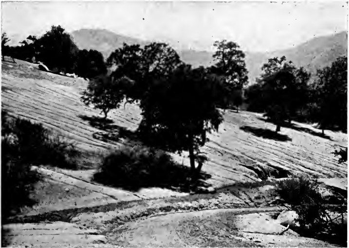
FIG. 131. — EROSION UPON AN UNPROTECTED SLOPE
