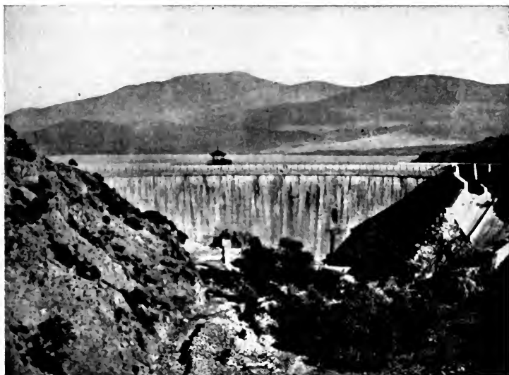
FIG. 116.—SWEETWATER RESERVOIR, NEAR SAN DIEGO, CALIFORNIA
