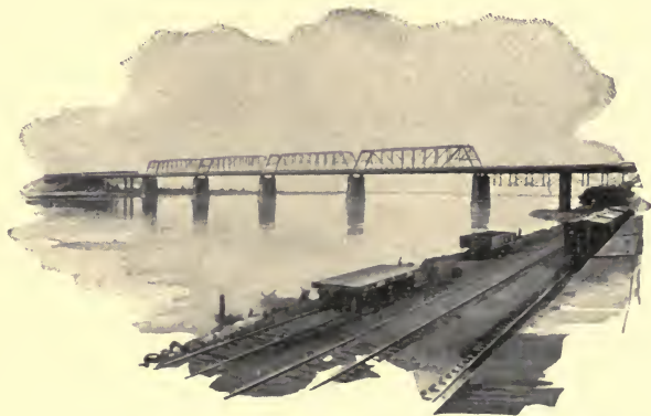
UNION PACIFIC BRIDGE ACROSS MISSOURI RIVER AT OMAHA.
