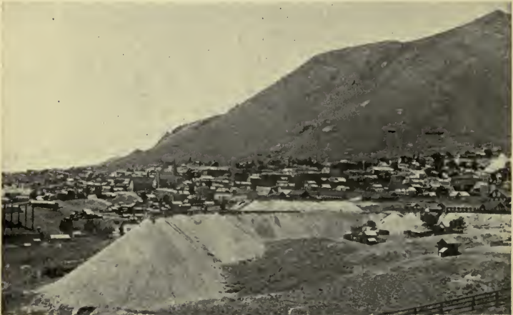
FIG. 120. — VIRGINIA CITY, NEVADA Supported entirely by mining
