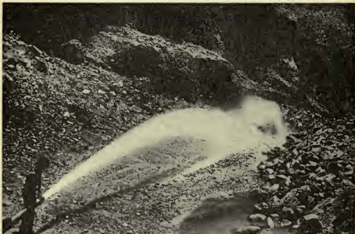
FIG. 100.—HYDRAULIC MINING ON THE KLAMATH RIVER, CALIFORNIA
