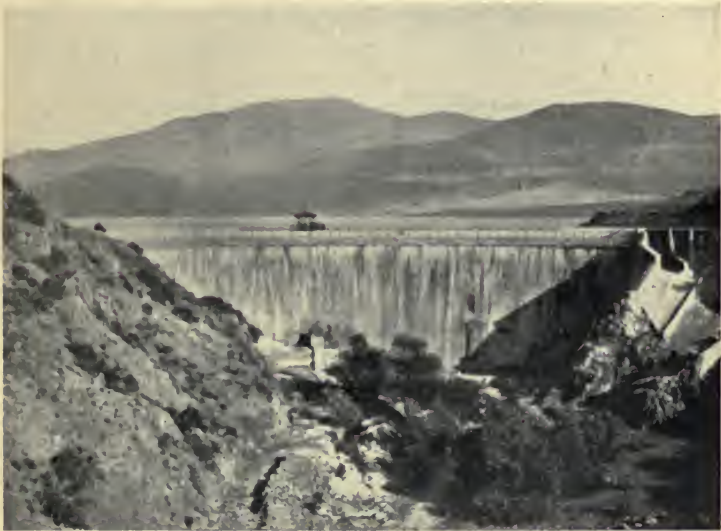
FIG. 116.— SWEETWATER RESERVOIR, NEAR SAN DIEGO, CALIFORNIA
