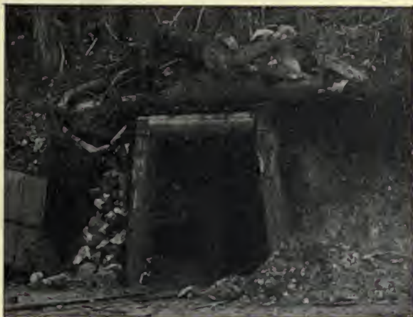
FIG. 98.—MOUTH OF A TUNNEL
