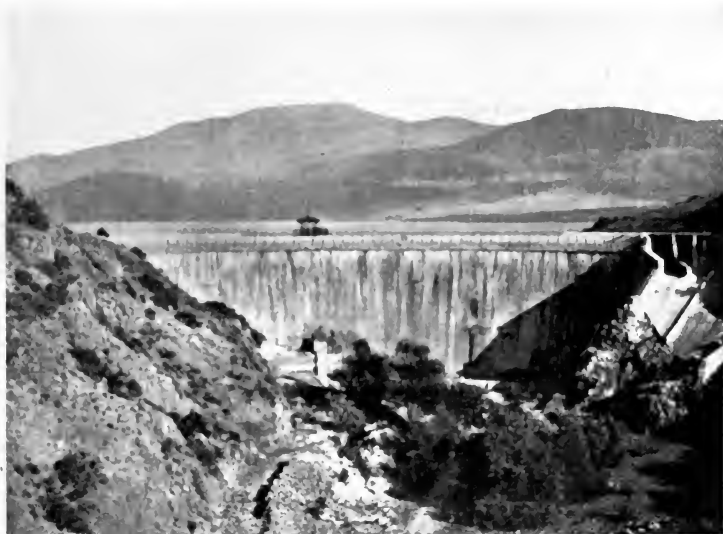
FIG. 116. — SWEETWATER RESERVOIR, NEAR SAN DIEGO, CALIFORNIA
