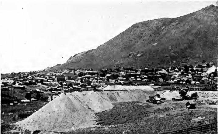
FIG. 120. — VIRGINIA CITY, NEVADA Supported entirely by mining
