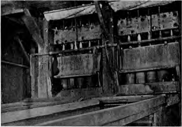
FIG. 103.—THE STAMPS IN A QUARTZ-MILL
