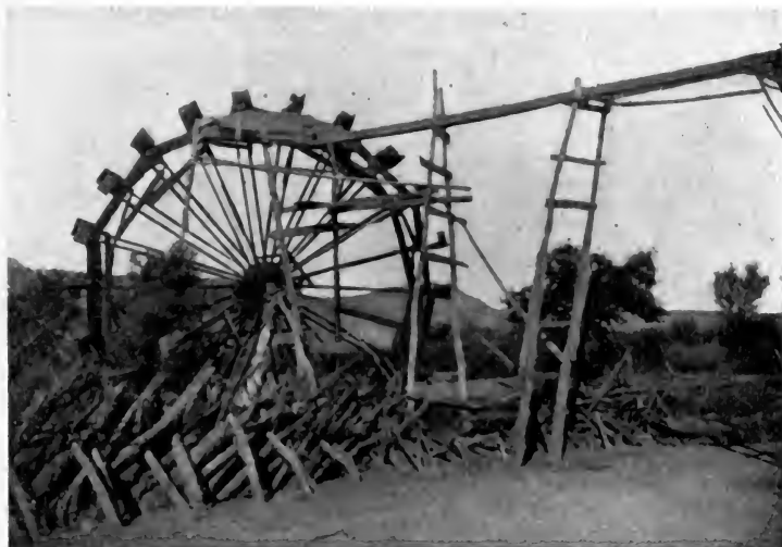
FIG. 113. — WATER-WHEEL FOR LIFTING WATER FOR IRRIGATION, VIRGIN RIVER, SOUTHERN UTAH
