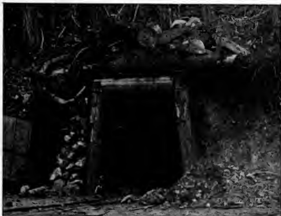
FIG. 98.—MOUTH OF A TUNNEL
