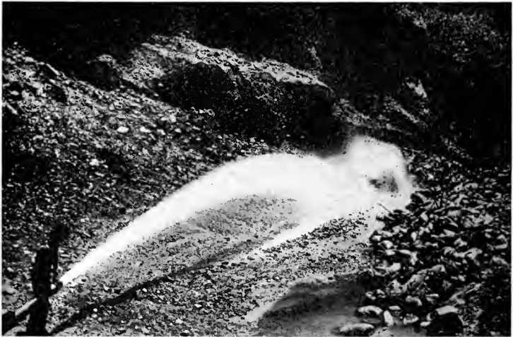
FIG. 100.—HYDRAULIC MINING ON THE KLAMATH RIVER, CALIFORNIA
