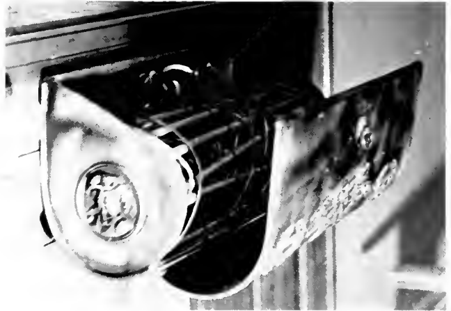
Utility made beautiful, a by-word of the day, exemplified in the hand-tooled red brass container for the wall mounted fire escape ladder from the third floor.
