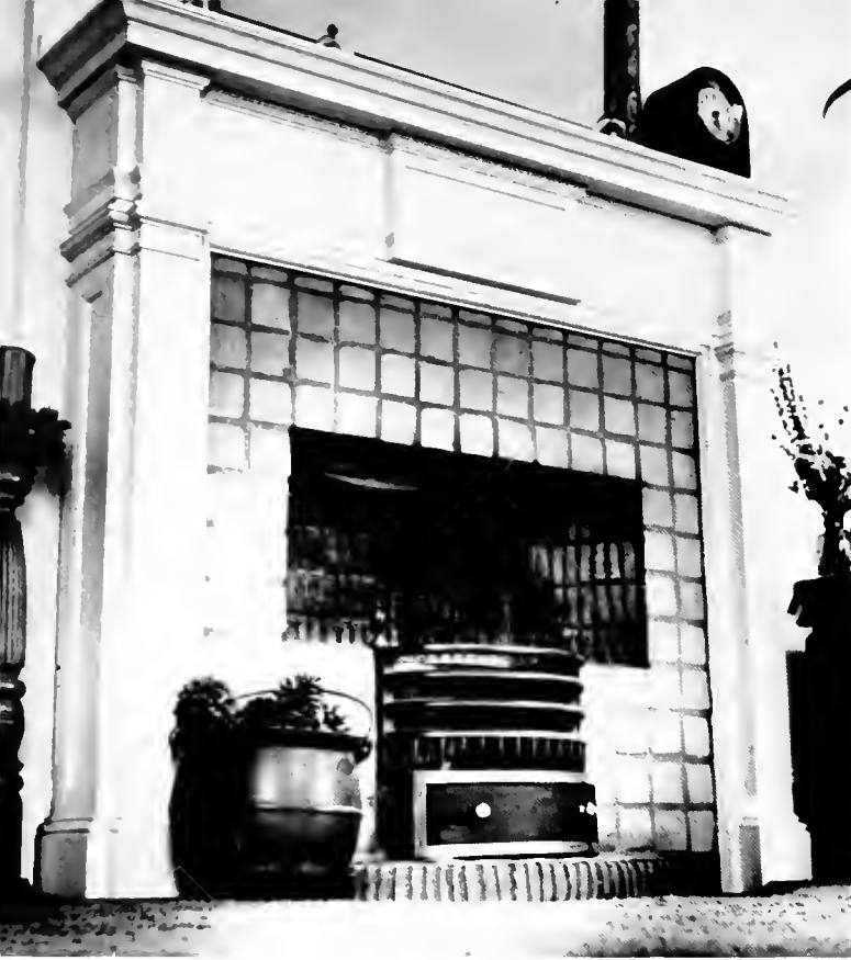
The second floor coal-burning fireplace features a curved drawer for the removal of ashes.
