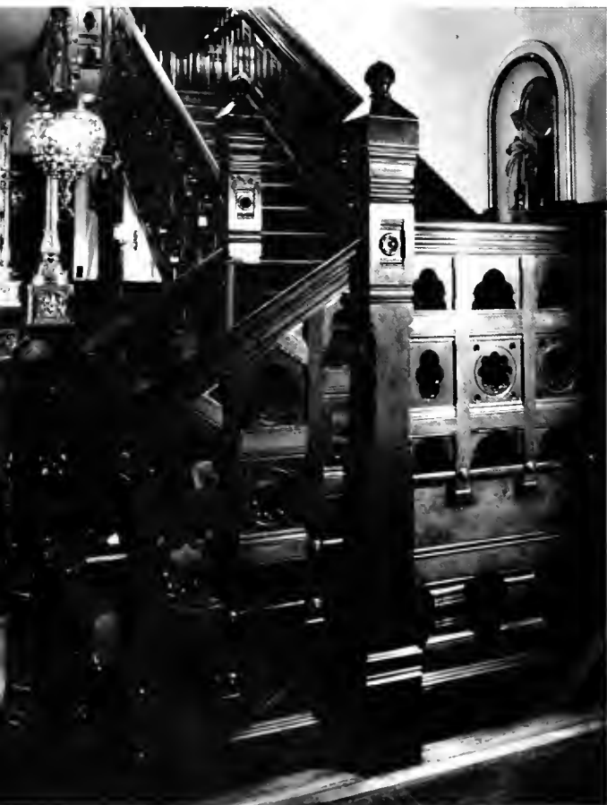
Newel post and gasolier detail.
