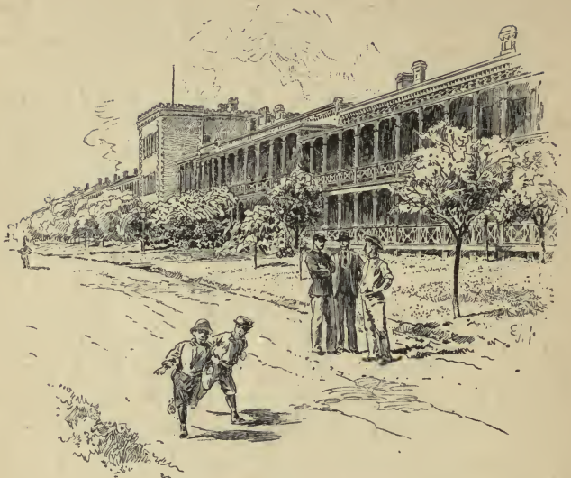
THE BARRACKS, FORT HOUSTON
