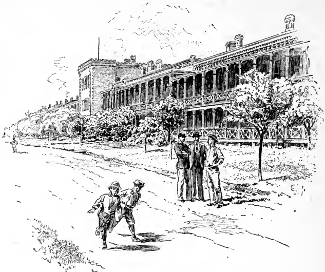
THE BARRACKS, FORT HOUSTON
