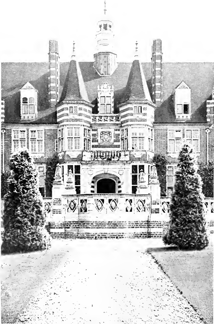
PLATE LXXVII.—S. JOHN'S SCHOOL, BEAUMONT: MAIN ENTRANCE AND TERRACE.
