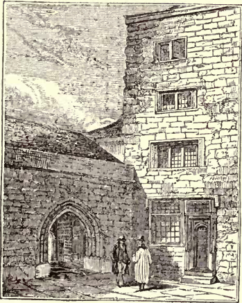
LITTLEINGTON TOWER IN 1840.
