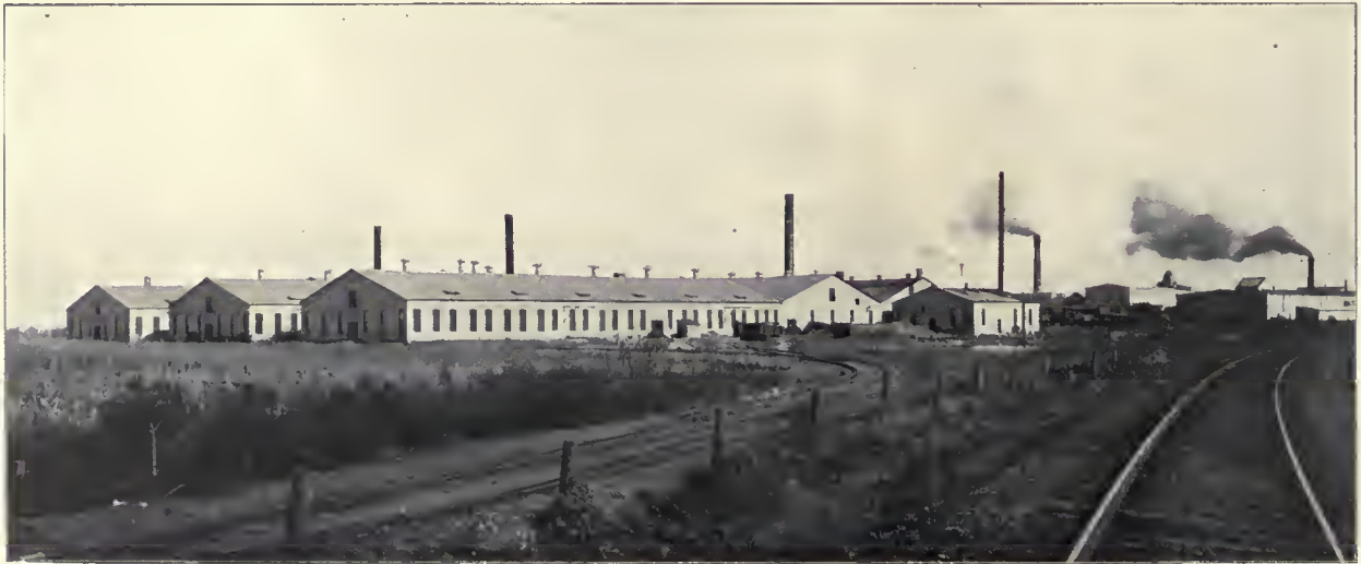
THE CHICAGO MALLEABLE CASTINGS COMPANY'S PLANT At 120th street and Center avenue. Established 1899. Covers 5\frac{1}{2} acres; 2 smelting furnaces of daily capacity of 12 tons each; 10 annealing ovens, capacity of 25 tons each. The Illinois Central tracks at the right, and the terminal tracks operated by the Chicago Terminal Transfer Company at the left.
