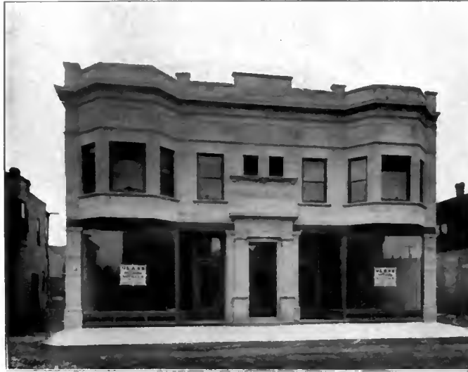
MARKET AND GROCERY STORE ON 120TH STREET Completed November, 1900
