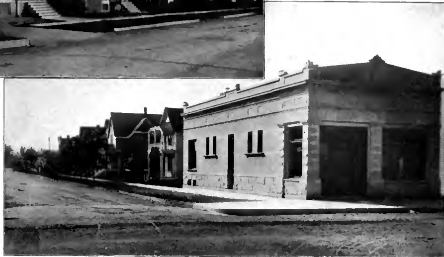
STATE BANK OF WEST PULLMAN At corner of 120th street and Lowe avenue. Bank established 1894. New building erected 1900.
