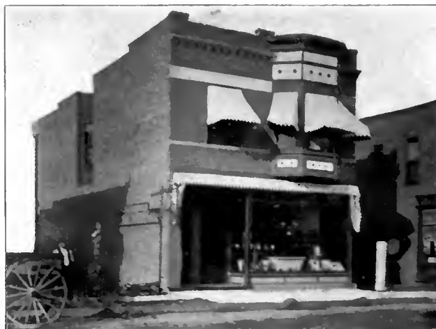
PLUMBER'S STORE, on 120th Street.
