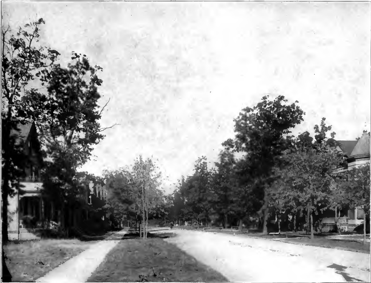
EGGLESTON AVENUE Looking north from 120th street
