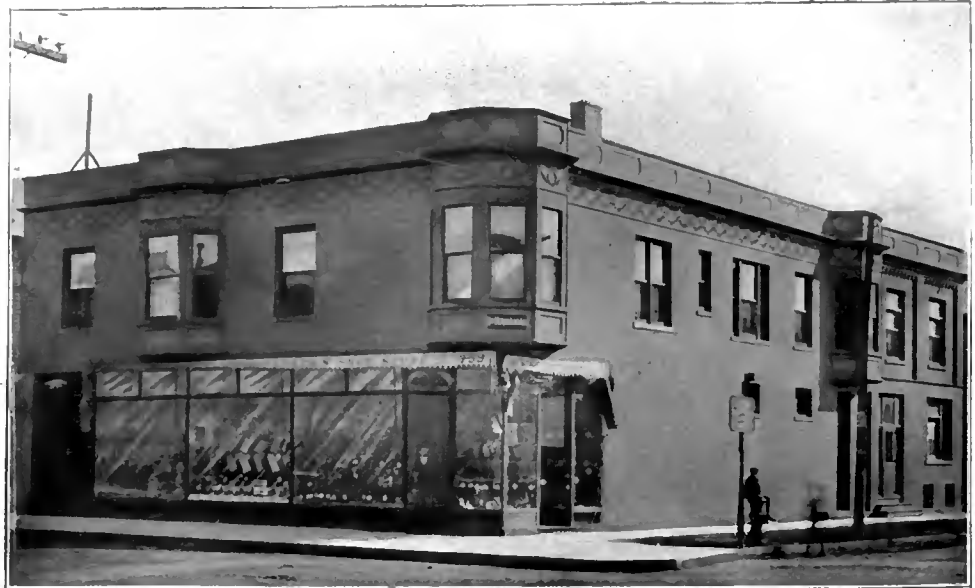
BRANCH OF CHICAGO PUBLIC LIBRARY, LOCATED IN THIS BUILDING, GIVING DAILY DELIVERIES.
