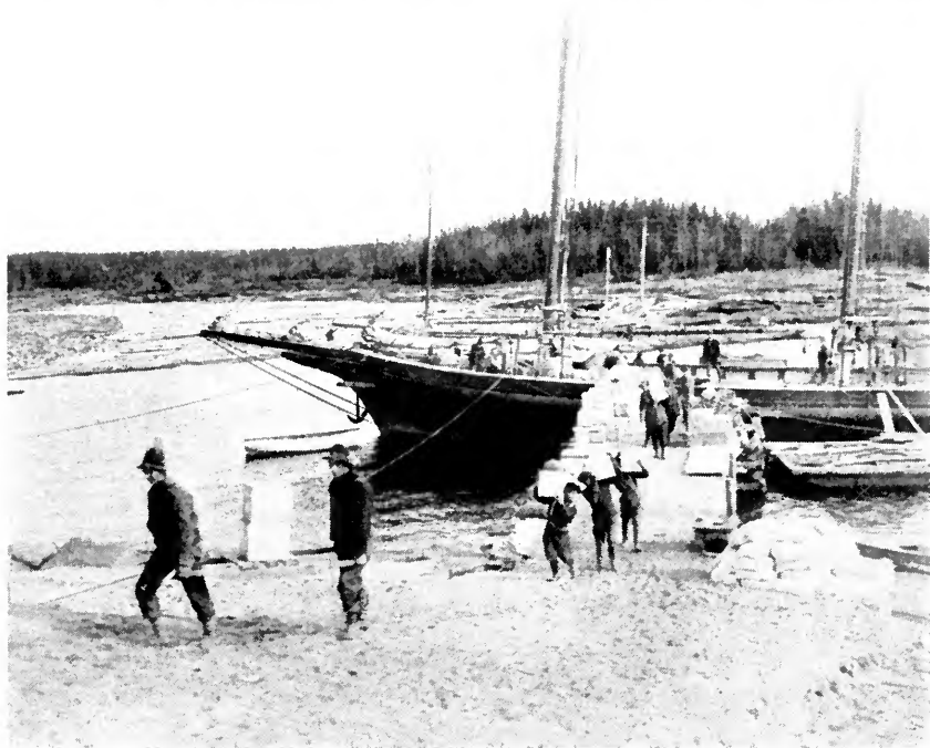
UNLOADING supplies from schooner in Rocky River at Shelter Bay.
