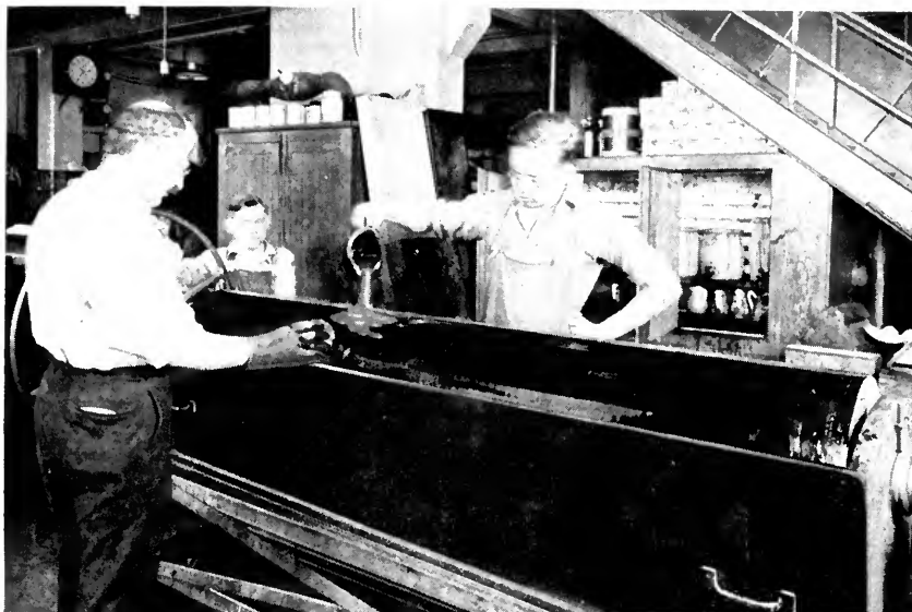
ETCHING one of the copper cylinders which print COLORoto.
