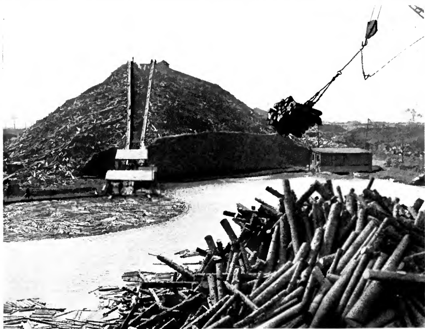
Logs lifted from the deck of a steamer are thrown into the pond at The Tribune's paper mill. They are floated across the pond and then built up into the huge storage pile.
