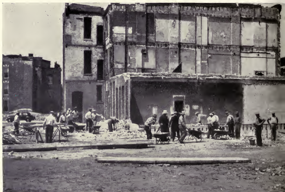
Demolition of slums goes ahead on two sites, in Chicago and Syracuse. This is Chicago's fourth low rent housing project, first for Syracuse.
