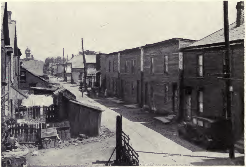
Splintering wooden buildings in Charleston, S. C., and Columbus, Ohio. New low-rent housing, soundly built and permanently protected from blight, will arise in both areas on the sites shown in these photographs.
