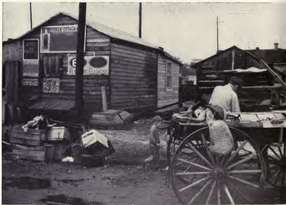
Meeting Street Manor, Charleston, shows how simple, orderly planning can result in a pleasant neighborhood. Below: chaos on the site of low-rent project now under way in Mobile.
