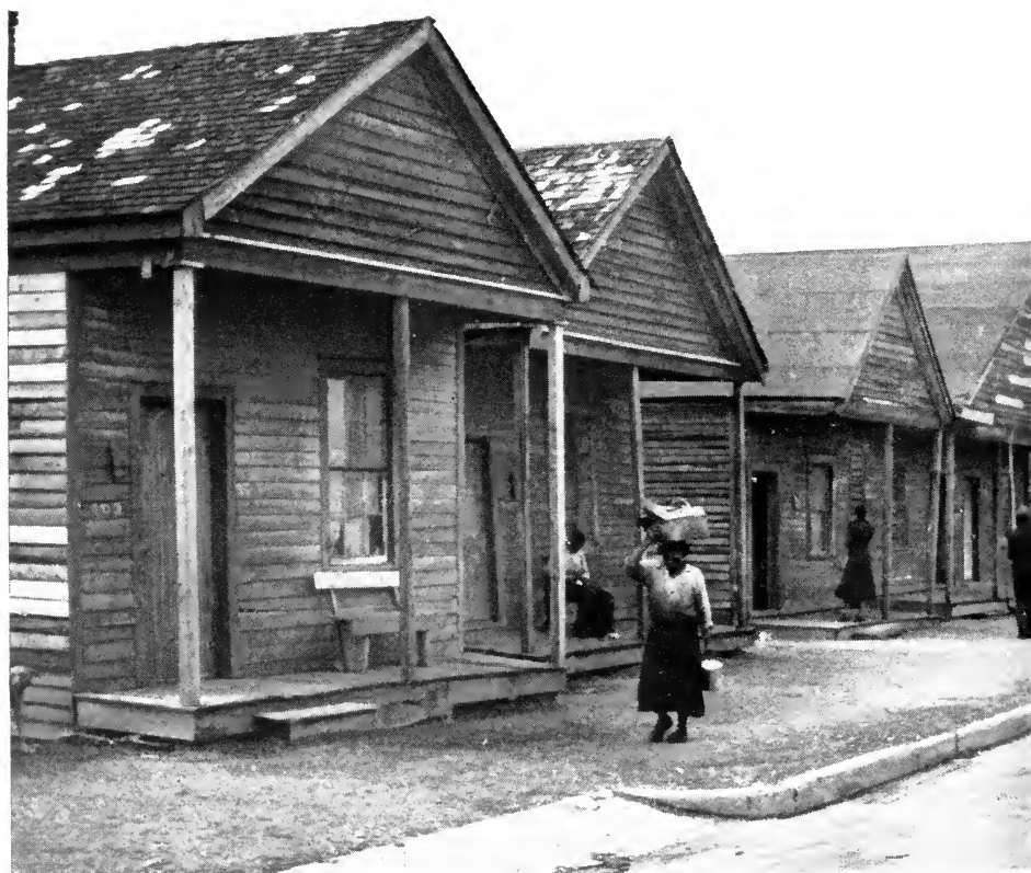
Substantial fireproof homes will replace these jerrybuilt houses in Youngstown, Ohio, (above) and Mobile, Alabama.
