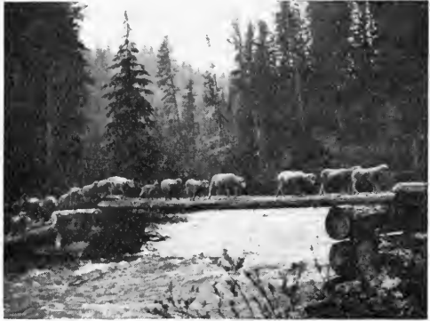
SHEEP BRIDGE ON THE DEADWOOD RIVER
