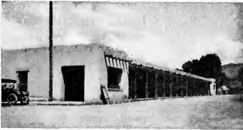
OLD PALACE AT SANTA FÉ
