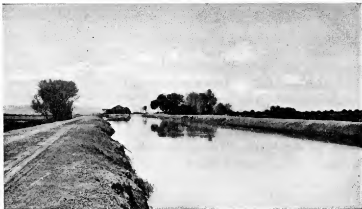
SALT RIVER PROJECT CANAL
