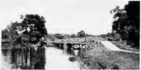
MORRIS CANAL TOWING BRIDGE ACROSS ROCK-AWAY RIVER
