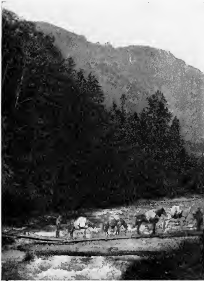
A PRIMITIVE BRIDGE IN SKAGIT COUNTY
