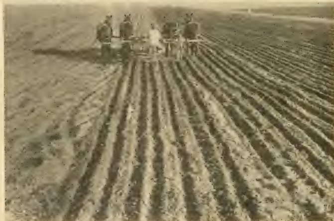
Fig. 12.—Late fall cultivation of summer fallow with twelve shovel, two-row corn cultivator to conserve moisture and prevent drifting.
