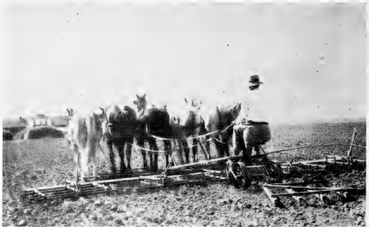
Fig. 19.—With a gang of harrows one man can cover eighty acres a day.
