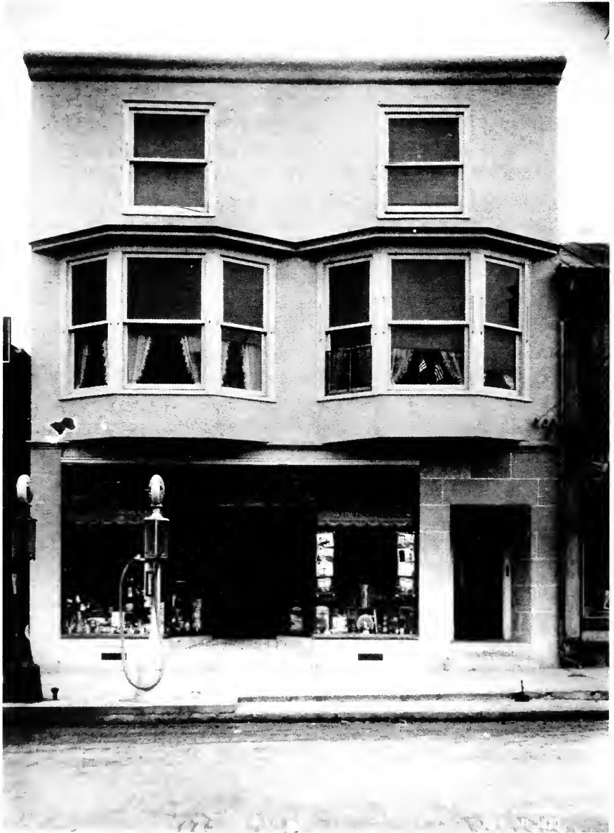
Fire destroyed the original general store in this Main Street building belonging to the Gudykunst family. After the turn of the century it was restored and became Frey's hardware.
