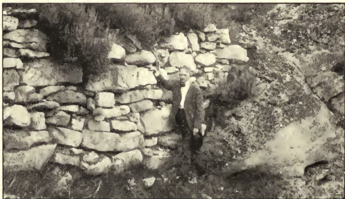
Part of fortifications built by Utah troops to hold back Johnston's army.
