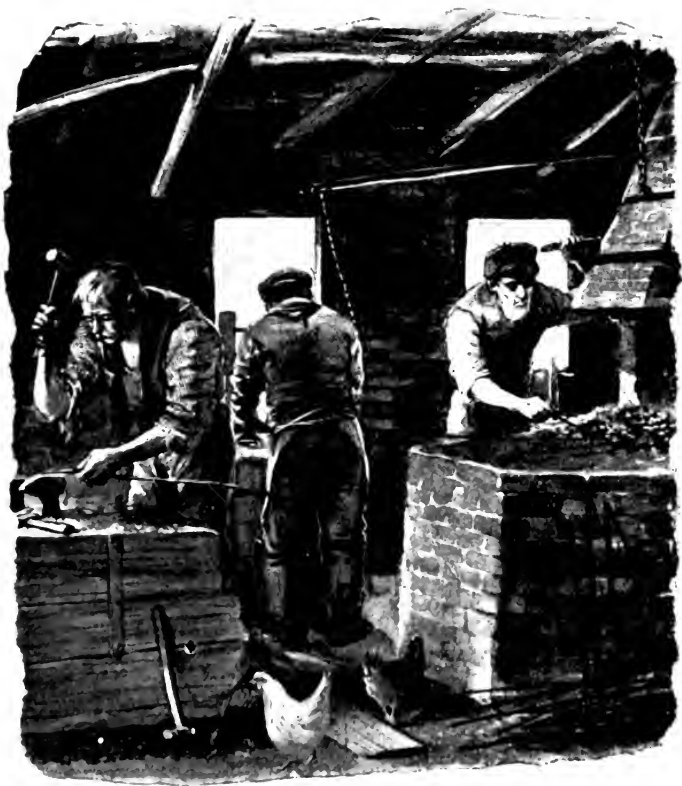
INTERIOR OF A BROMSGROVE NAILMAKER'S SHED, OCCUPIED BY THE TENANT AND TWO STALLERS, THE LATTER WORKING EACH ON HIS OWN ACCOUNT, AND PAYING 6d. A WEEK APiece AND ONE-THIRD OF THE FIRING. THE OLIVER, OR HEAVY HAMMER USED FOR HEADING THE NAILS, IS ATTACHED TO THE BENCH IN FRONT OF THE LITTLE ANVIL.
