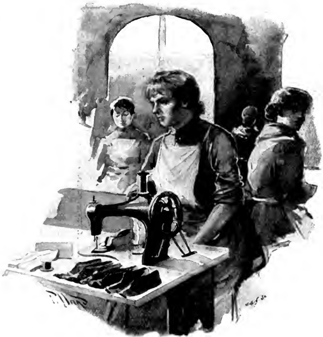
FITTING TOE-CAPS TO SLIPPER-TOPS.
