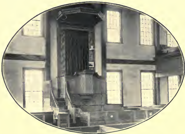
INTERIOR OF ROCKY HILL CHURCH
