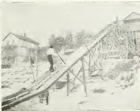
8.—CONVEYING ICE BLOCKS UP THE CHUTE.—THIS IS VERY DANGEROUS WORK. From a Photo. by the Author.
