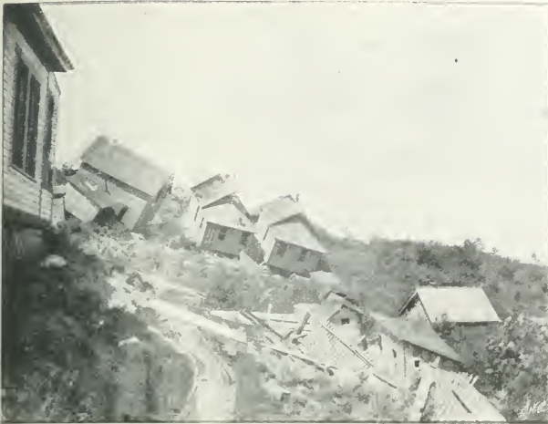
11.—PART OF THE SUBURBS OF SEATTLE CITY SLIDING DOWN INTO LAKE WASHINGTON. (From a) (SPEED, ABOUT \frac{1}{4} IN. PER DAY.) (Photo.)
