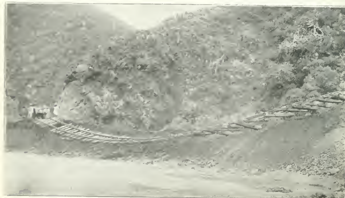
14.—HOW FLOODS LEAVE THE PERMANENT WAY OF THE MEXICAN SOUTHERN RAILWAY. [Photo.]
