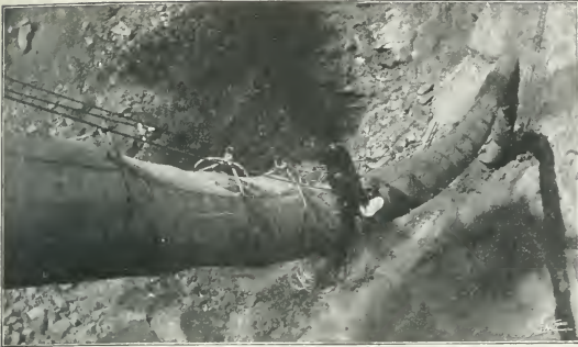
HERE WE SEE THE MEN PREPARING TO SEND DOWN CARBONIC ACID GAS TO From a) EXTINGUISH THE FIRES. STEAM AND SAND WERE ALSO TRIED. [Photo.]
