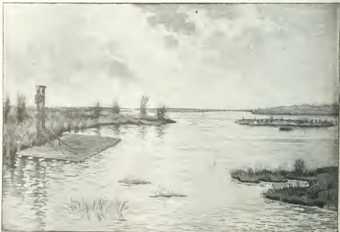
WHEN THE ISLANDS WERE CAPTURED, THEY HAD TO BE KEPT PRISONERS BY MEANS OF LINES OF STAKE-PILE-DRIVING HAMMER ON LEFT.
