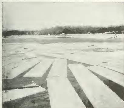
6.—HERE ARE THE ICE SLABS READY FOR GLIDING TO THE TROUGH. From a Photo. by the Author.
