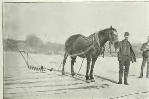
1.—THIS IS THE ICE-PLOUGH BY MEANS OF WHICH THE ICE SURFACE IS DIVIDED INTO SQUARES. From a Photo. [by the Author.]
