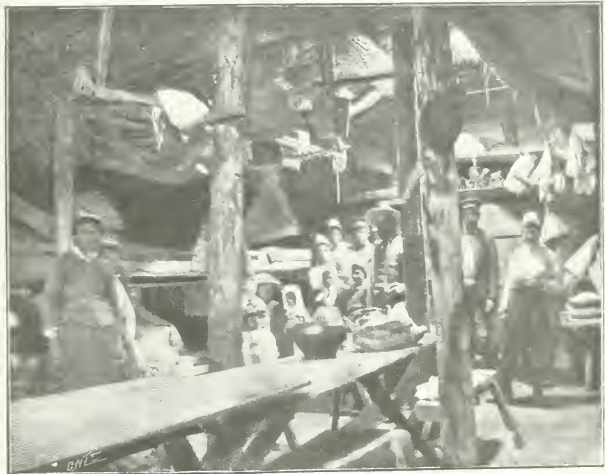
FIGURE 1. INTERIOR OF A DWELLING BUILT BY THE WONDERFUL DOUKHOBOR HOUSES. [Photo.]
