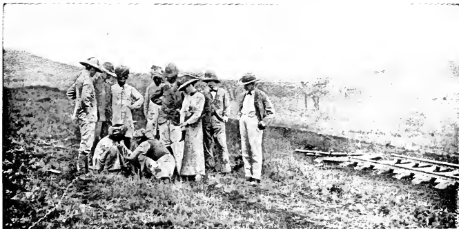
GROUP OF MISSIONARIES, ETC. WATCHING TWO INDIANS JOINING THE ENDS OF THE TELEGRAPH LINE ON THE UGANDA RAILWAY. [Photo.]
