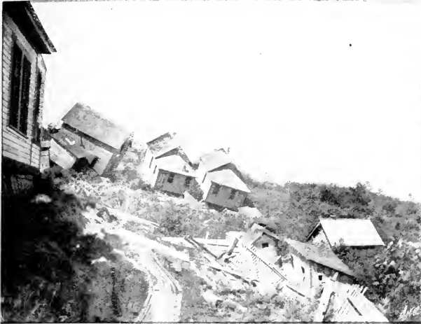
11.—PART OF THE SUBURBS OF SEATTLE CITY SLIDING DOWN INTO LAKE WASHINGTON. (SPEED, ABOUT 2½ IN. PER DAY.) (Photo.)
