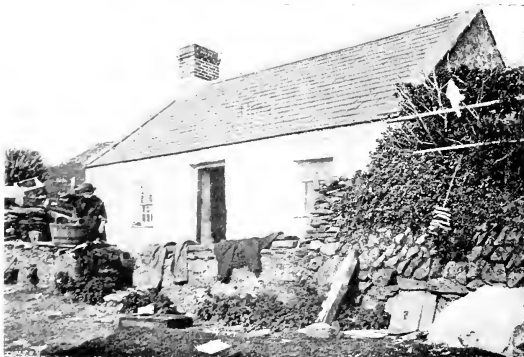
THE HOUSE OF THE OWNER. From a Photo. by Milton, Poldheli.
