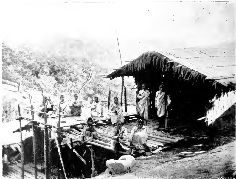
THE LUSHAI HOUSE. "THEY LOVE TO PERCH THEIR HOUSES ON THE HIGHEST PEAKS AND LOOK DOWN UPON THE CLOUDS." (By the Authors.)
